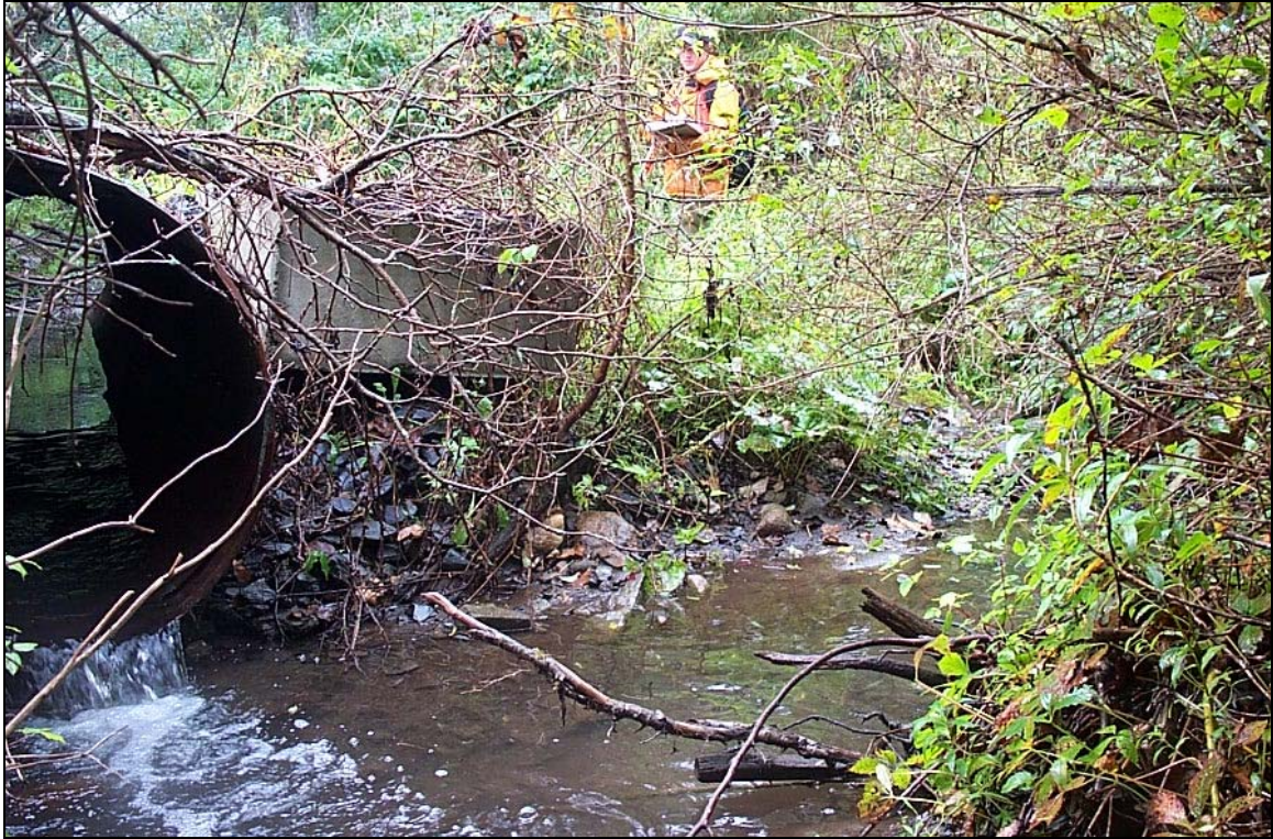
Figure 36: Undersized culverts disrupt the sediment transport capacity of the stream and may lead to both upstream and downstream destabilization. Improperly sized structures, such as this one on T3.01-A, can become plugged and lead to a channel avulsion.
