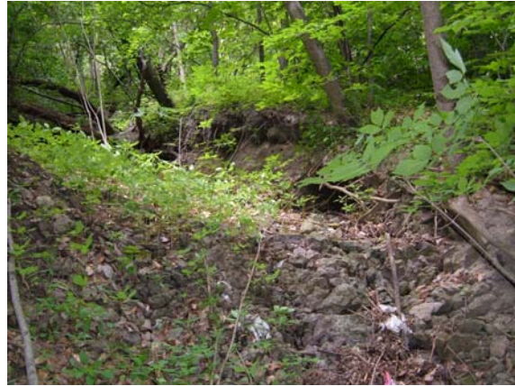
Figure 4. Gully in lower T2.02-A
