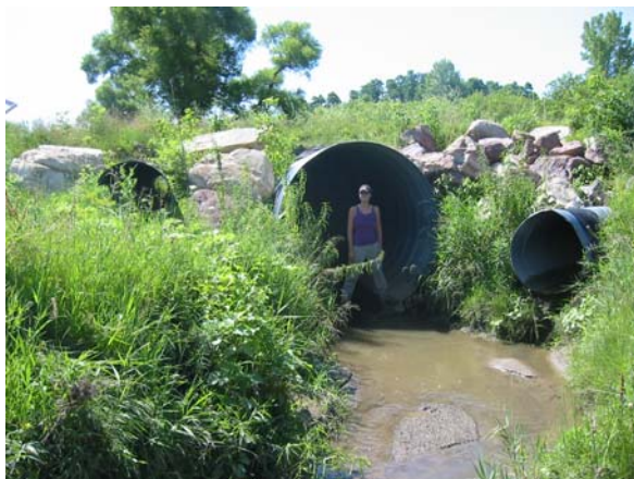
Figure 4. Culvert crossing midway through reach M02-A
