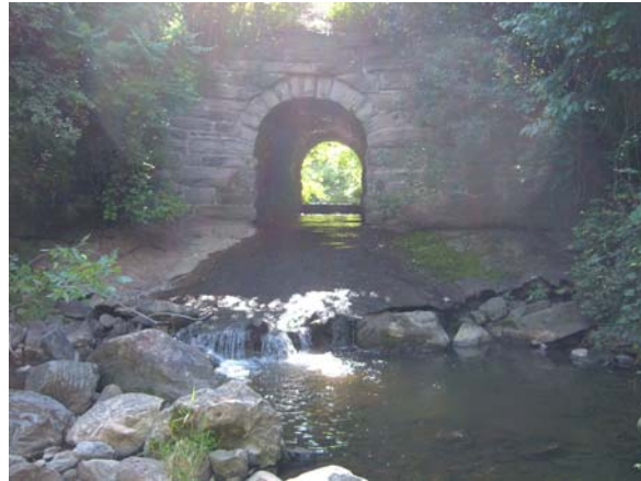
Figure 2. Railroad crossing grade control mid-reach
