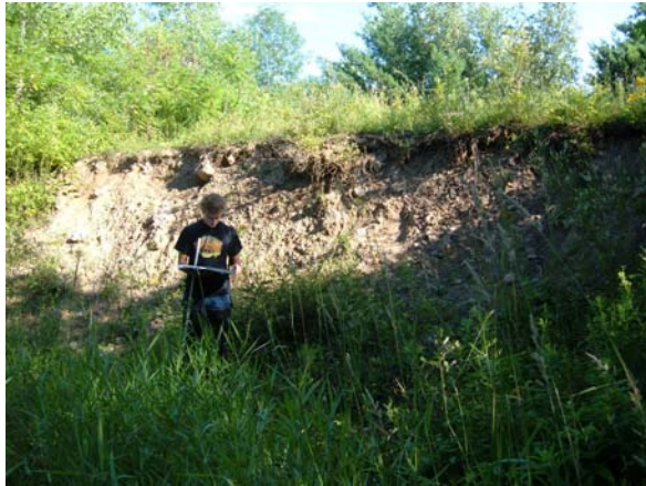
Figure 1. Mass failure on flood chute in reach M01
