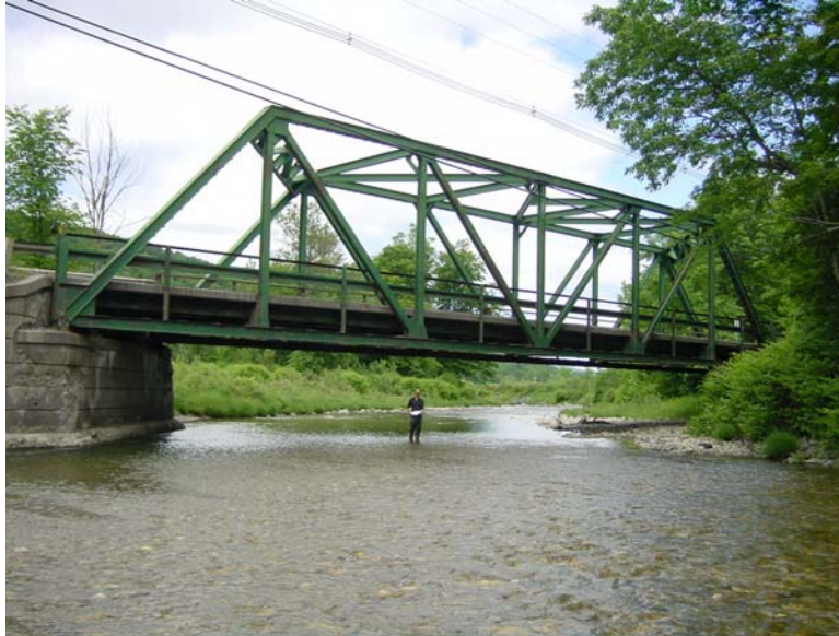
Figure 6.22 Warren Trestle Bridge
