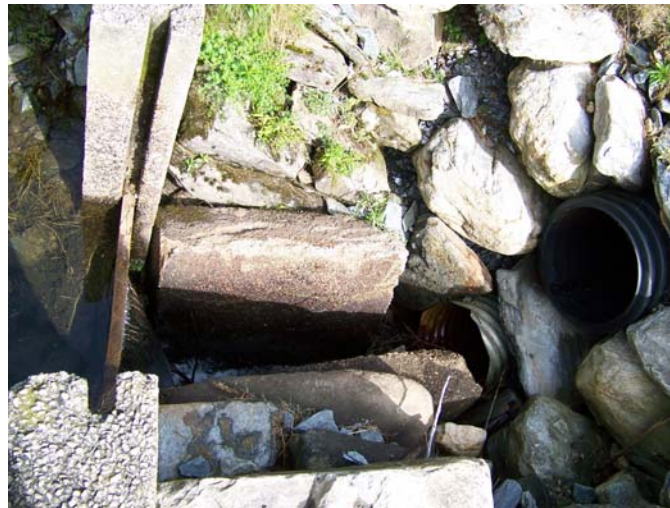
Figure 6.2 Culverts under part of the golf course on T9.3S1.01. A dam is seen on the left then 2 small culverts on right that travel under the golf course.
