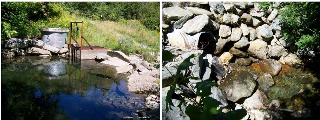
Figure 6.5 A dam and culvert on T9.04 adjacent to the ski area. The photo on the left is an upstream view with a dam and pond. The right photo shows the downstream view with a pool and riprap.
