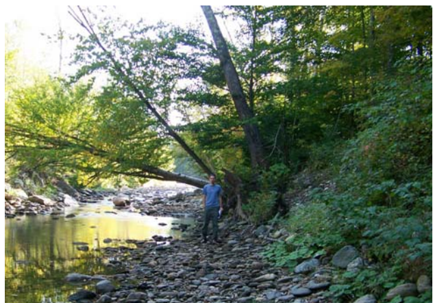
Figure 6.30 Bank erosion above Route 100 bridge.
