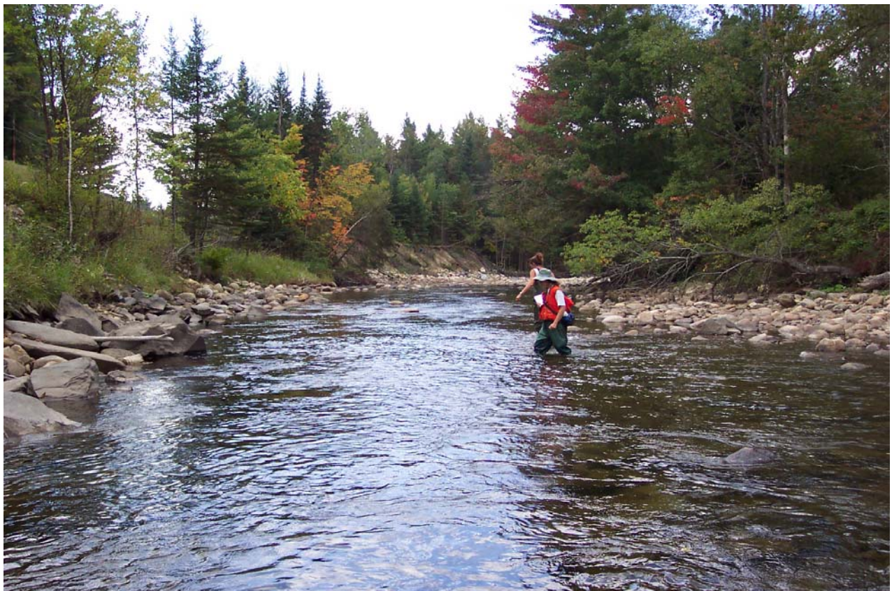
Figure 27: Reach T103 with Route 114 on left, mass failure downstream and floodplain pockets along right bank, photo taken in 2003 one year after flood
