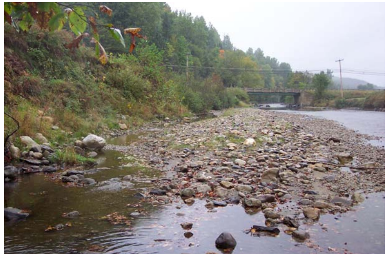
Figure 20: Looking upstream towards Route 114 Bridge on Reach T102B, Riverside Center on left. Sediment deposits and channel widening evident.
