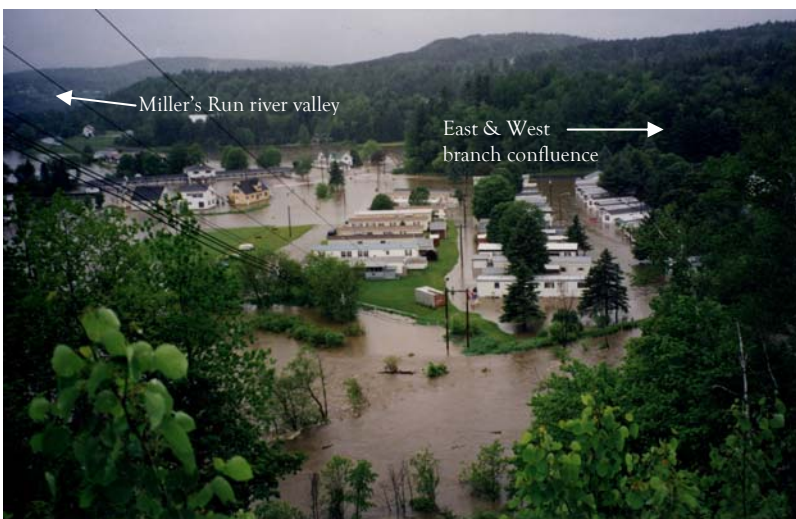
Figure 2: Photo by Kenneth Mason: 2002 Passumpsic River main stem flooding near junction of Rte 114 and Rte 5 in Lyndon and Miller's Run confluence
