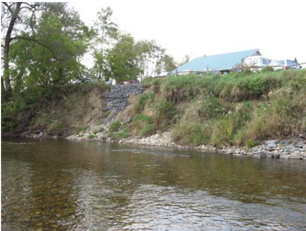
Figure 13: Right bank of Reach T101B showing streamside residence and business that could be impacted by fluvial erosion hazards. Tall eroding banks also observed showing poor access to floodplain.
