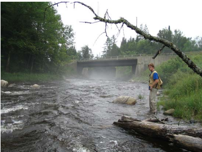
Figure 42: Reach T107B Route 114 90' wide bridge with 35' old abutment immediately downstream
