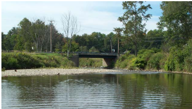
Figure 12: Photo taken in 2003, one year after flood, looking downstream towards Lily Pond Bridge on Reach T101A. Bridge is a channel constriction, showing sediment accumulations upstream, and was an area of conflict during flood.
