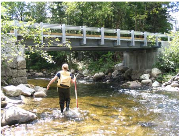
Figure 41: Reach T107B Worden Road Bridge
