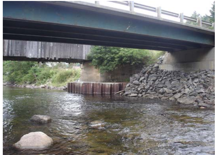
Figure 17: View looking downstream beneath Burrington Bridge covered bridge in background on Reach T102A taken in 2009. New footing on covered bridge and additional rock placed under Burrington Bridge.
