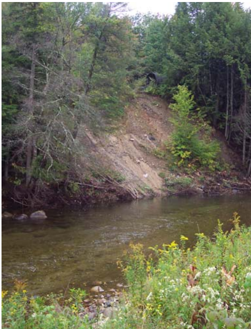
Figure 19: Mass failure on Reach T102B
