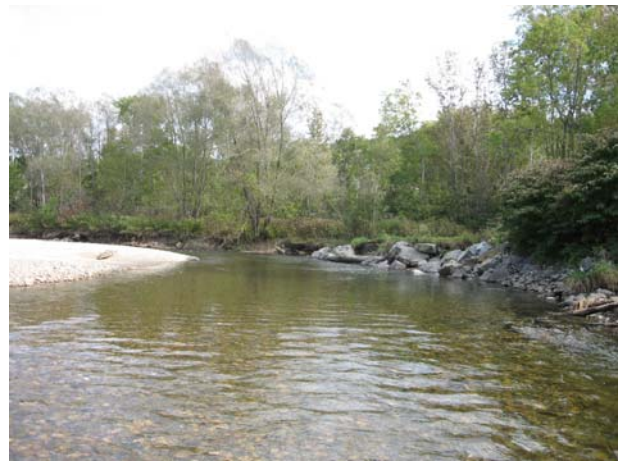
Figure 14: Reach T101B looking upstream showing new bank armoring protecting residential activities along left bank. Some new bar development on opposite bank
