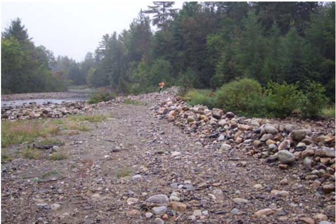
Figure 23: Looking upstream at berm on Reach T102C in 2003, one year after flood.
