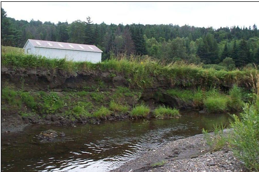
Figure 9. Extensive lateral bank erosion on outside bends in reach M03.
