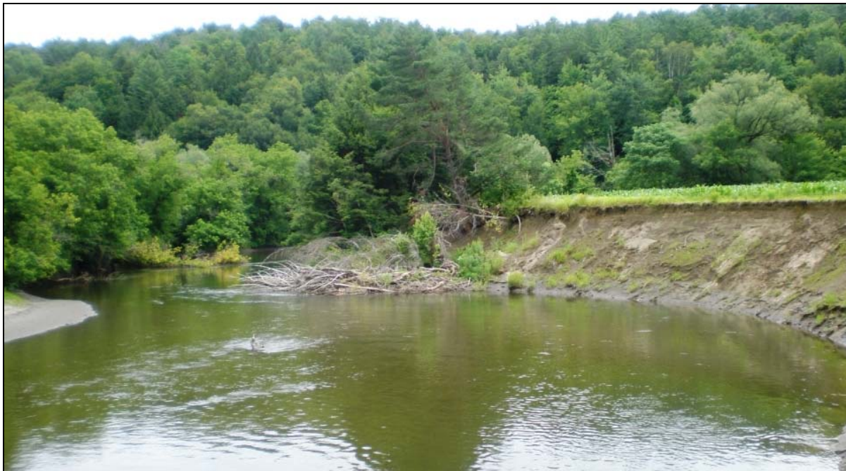
Figure 9: Significant streambank erosion through alluvial soils in reach R23.
