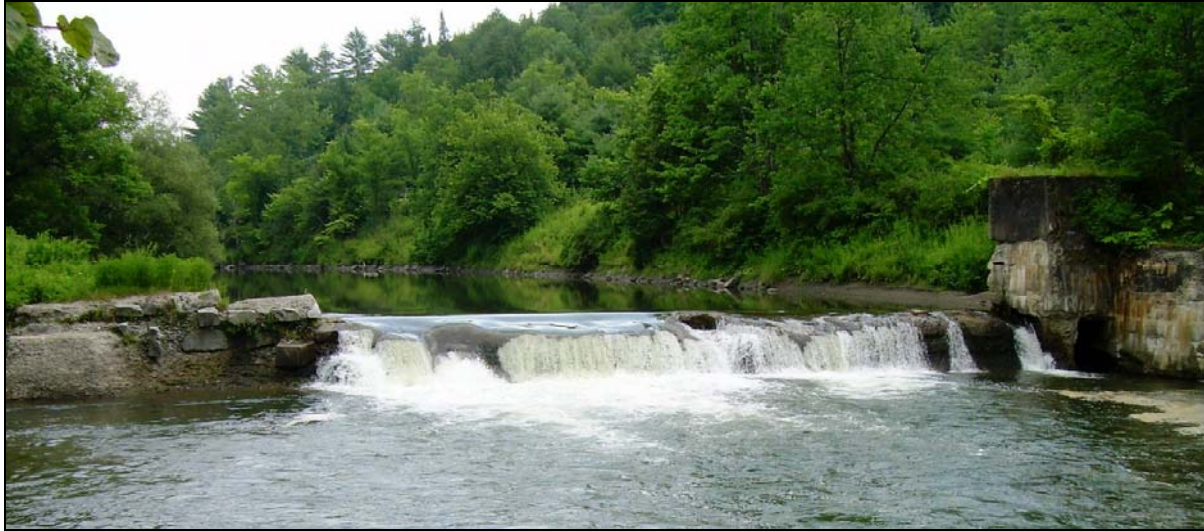
Figure 15: An old concrete dam disrupts water and sediment transport at reach R21-A (looking upstream).
