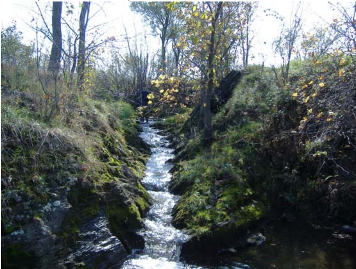
Figure 3 Channel Spanning Bedrock M4T2.03
