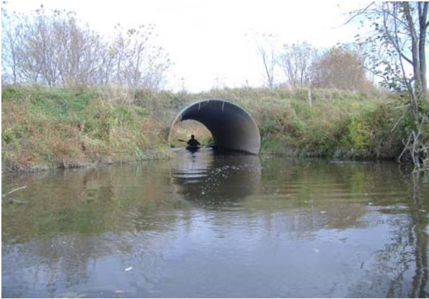
Figure 22 Heald Road culvert M3T1.01
