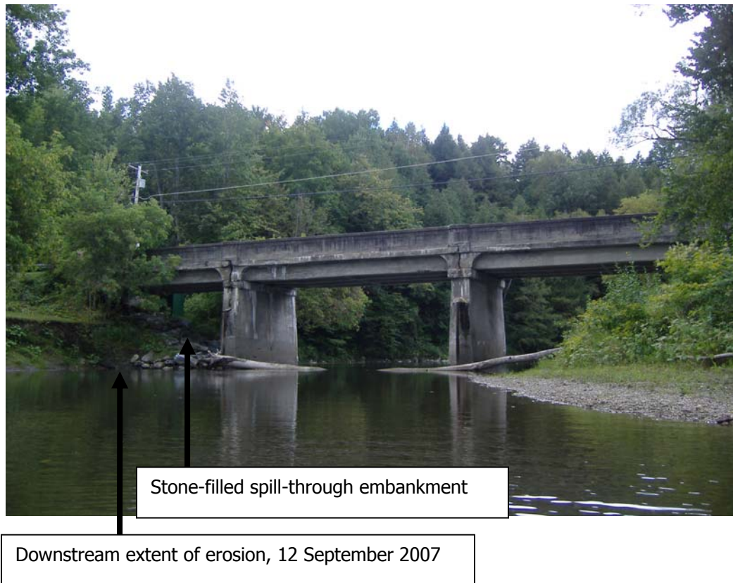
Figure 14. Site of LB erosion upstream of Dog Team Road bridge, reaches M01 and M02. (View downstream to the bridge, 12 September 2007).
