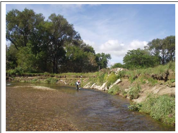
Figure 37. Less than 5-foot riparian buffer along an eroding meander in reach M04. Buffer in this location is dominated by grasses which provide little root-binding capacity to streambank soils and negligible shade to the river channel.
