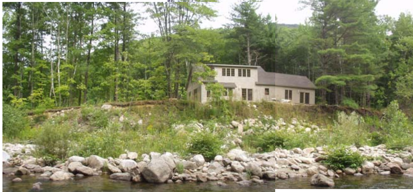
Figure 26. Newly-constructed home located within 10 feet of the top of an actively eroding sand and gravel stream bank. Reach M15, right bank. Rockydale, Bristol, VT.
