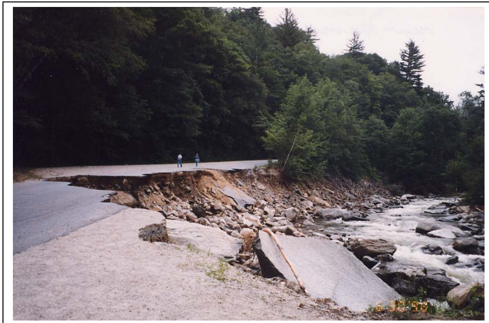
Photo 6. Bristol / Lincoln Road washout, 1998 flood. Just downstream of Bartlett's Falls. Susan Tucker collection.
