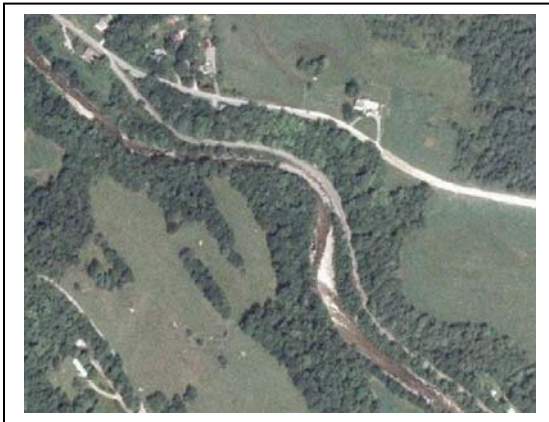
Figure 9. Example of local reduction in sediment transport capacity, Reach M18 along River Road just upstream of the Forge Hill Road intersection. Flow in New Haven River is from lower right on the image to upper right.
