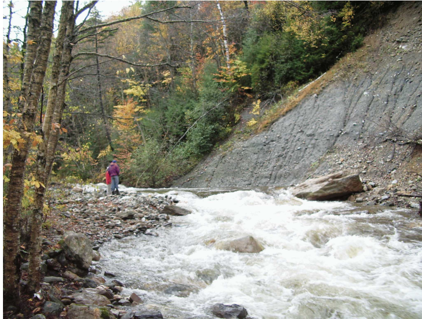
Figure 4. Landslide below Cooley Glen Bridge looking upstream from east bank
