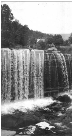
Large dam at bedrock exposures in the New Haven River at the former Grist Mill location along River Road southeast of Lincoln village and northeast of the Lincoln Community School (1909; Vermont Historical Society).
