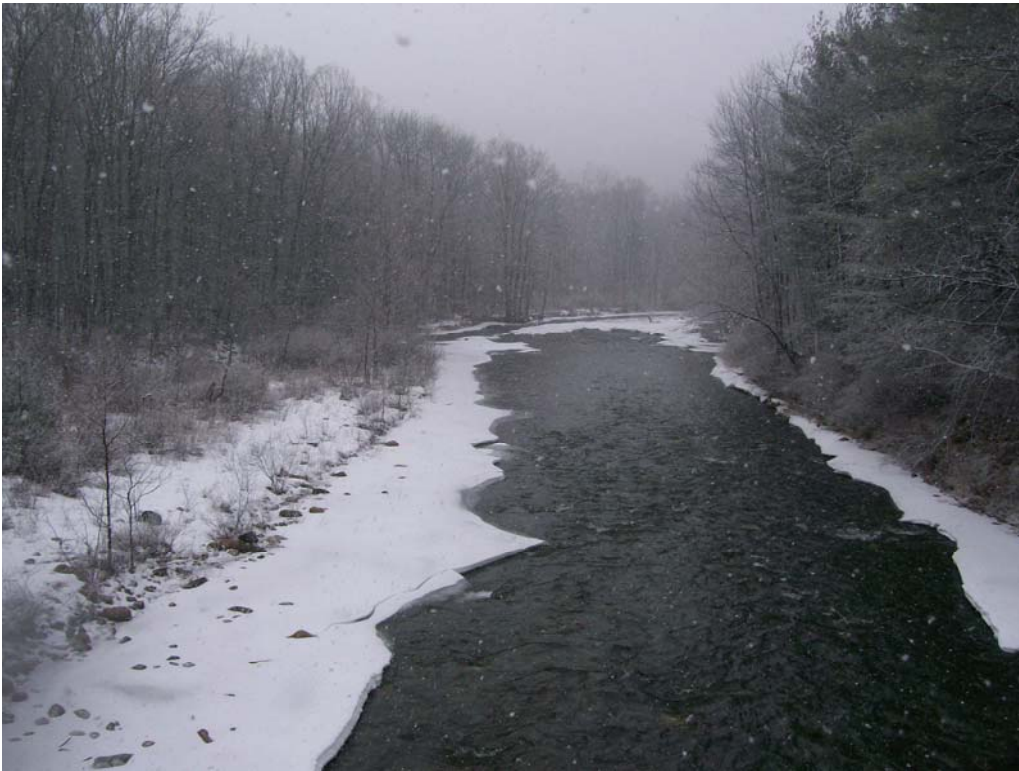
Figure F-1: Looking downstream from Route 7A Bridge. Large sidebar on left with upper left berm in background.
