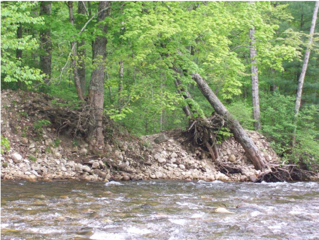
Figure F-24: Close-up of downstream end of lower left berm and erosion site.
