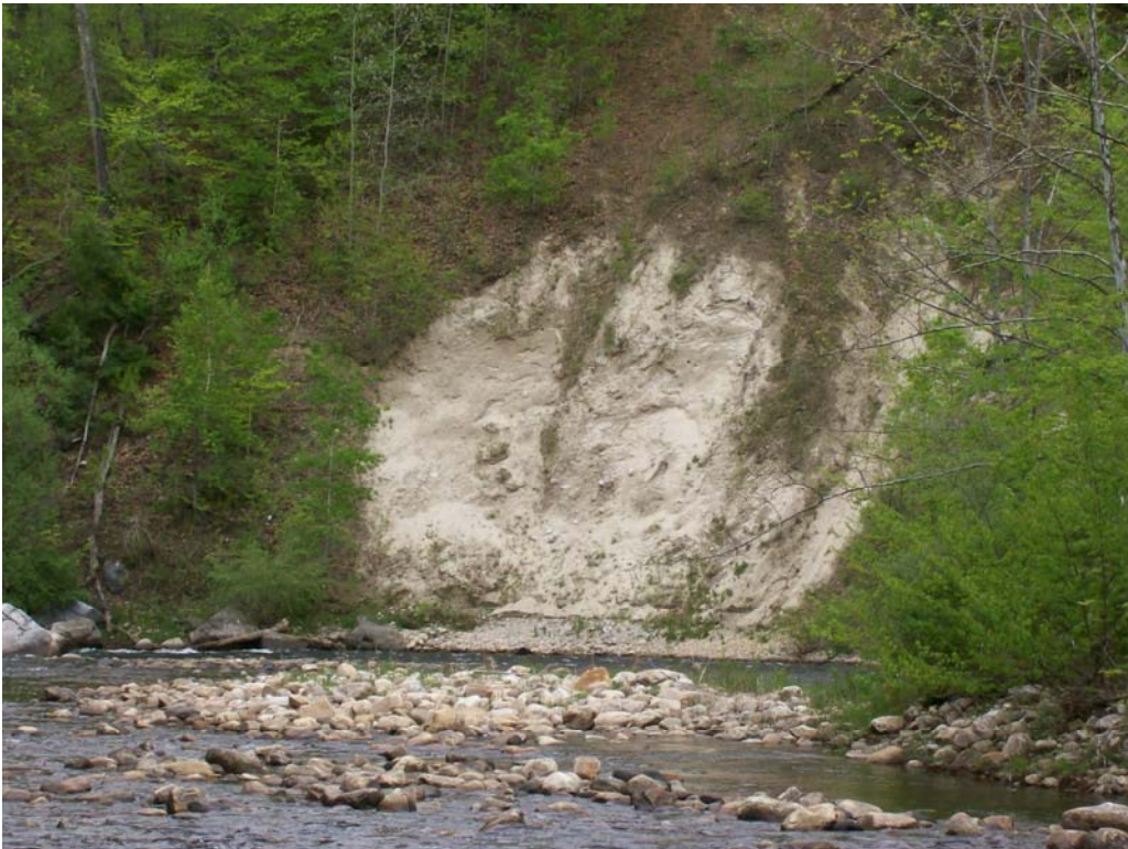
Figure F-26: Close-up of mass-failure site.
