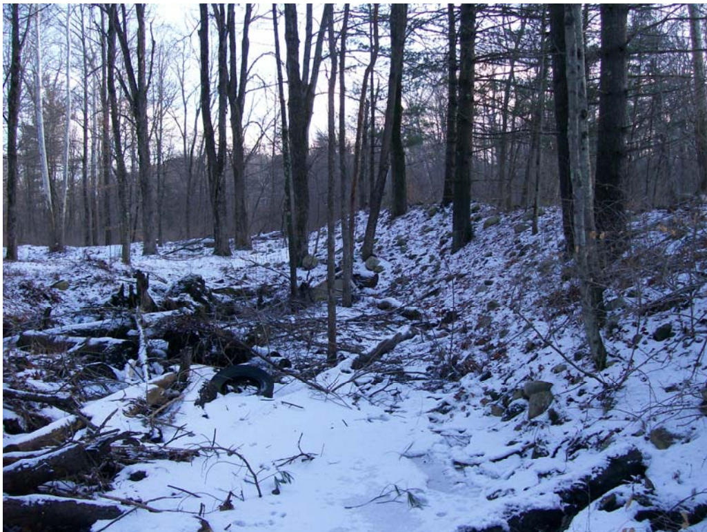
Figure F-20: Lower right berm viewed from right floodplain behind it looking upstream (note debris piled in low area).
