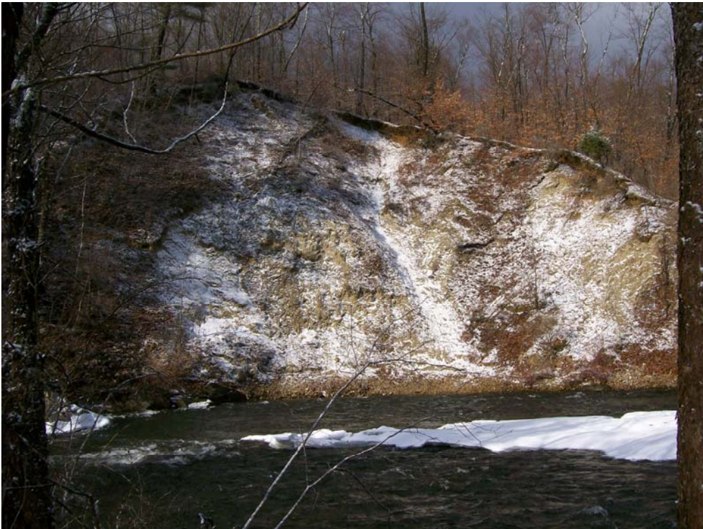
Figure F-14: Close-up of mass failure site.
