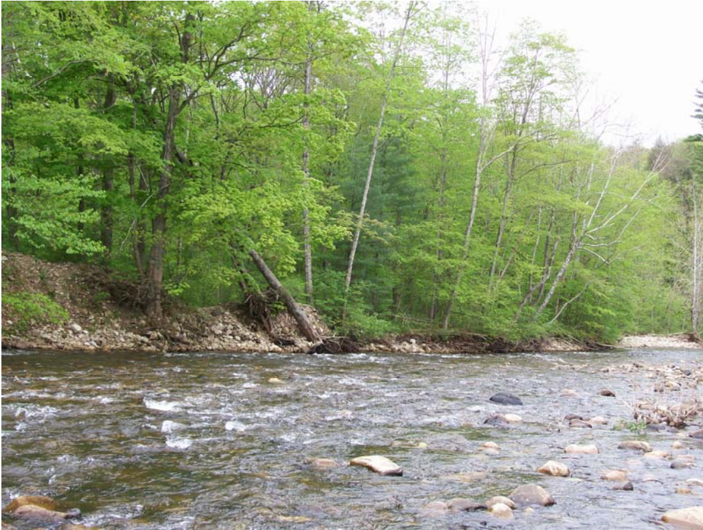
Figure F-23: Downstream end of lower left berm. Note erosion.
