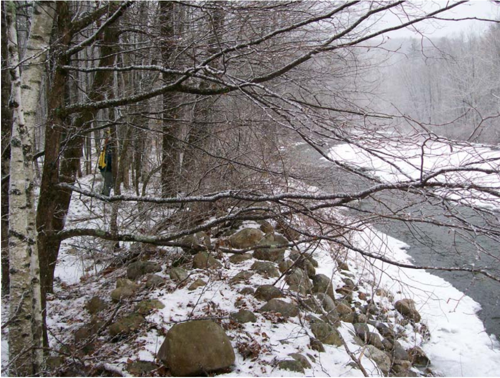
Figure F-7: Looking down upper left berm. Island in background.
