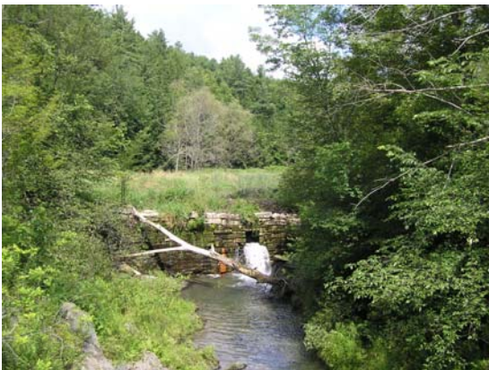
Figure 38. Pelletier dam is coincident with the downstream reach break for T02.09-s1.02. A wetland (former mill pond) is present upstream of the dam for a distance of approximately 400 feet. View upstream from East Hubbardton Rd bridge crossing.
