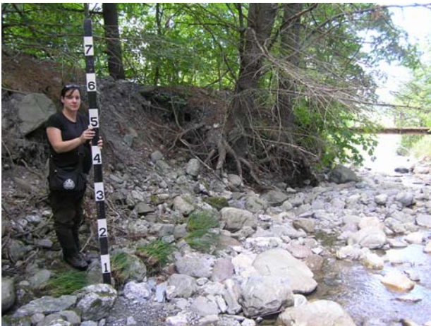
Figure 31. Gravel and cobble berm along left bank of Gully Brook upstream of Woodbury Road bridge crossing. Berm height ranges from 4 to 9 feet above channel thalweg.
