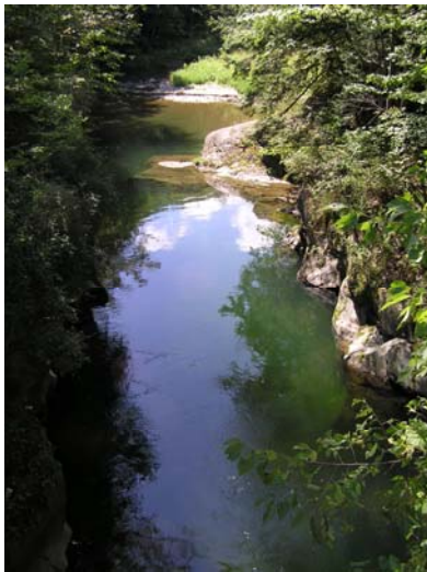
Figure 3. (M03) Bedrock gorge beneath Route 153 crossing at the Williams Bridge. This channel-spanning exposure of bedrock serves as a vertical grade control for the Mettowee River channel.
