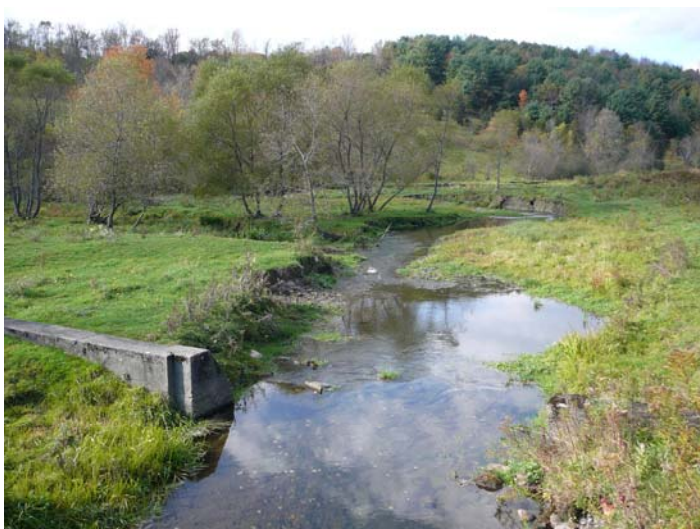
Figure 86. Possible dam structure at upstream end of Segment A of Indian River reach MNY10T1.07. View downstream through pasture, 13 October 2006.
