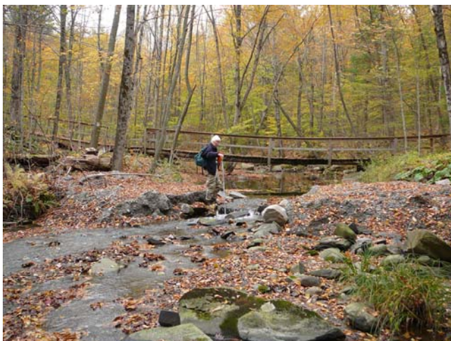
Figure 81. Small dam or possible ford of fine gravel and sand recently breached by flow in the channel within Segment B of Indian Brook, reach MNY10T1.08. View upstream, 11 October 2006.
