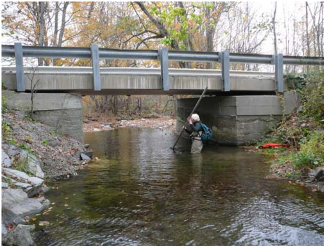
Figure 83. Sawmill Road bridge crossing in Segment E of Indian Brook, reach MNY10T1.07. View downstream, 11 October 2006.
