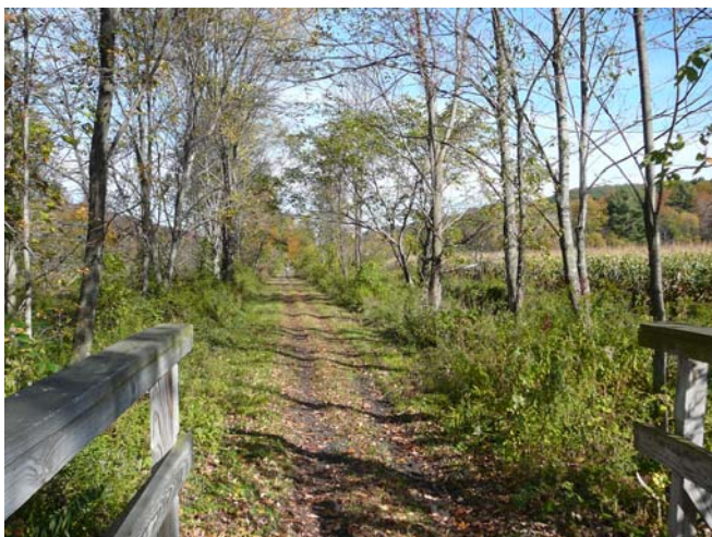
Figure 75. Rail trail crossing of Indian Brook in Segment A, reach MNY10T1.10. View to the north, 6 October 2006.
