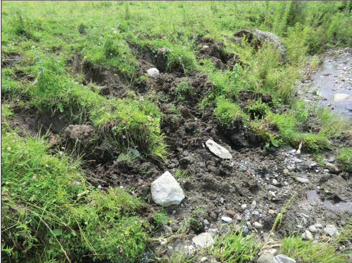
Figure 5.37. Animal access in M06S3.01-C is contributing to bank instability.
