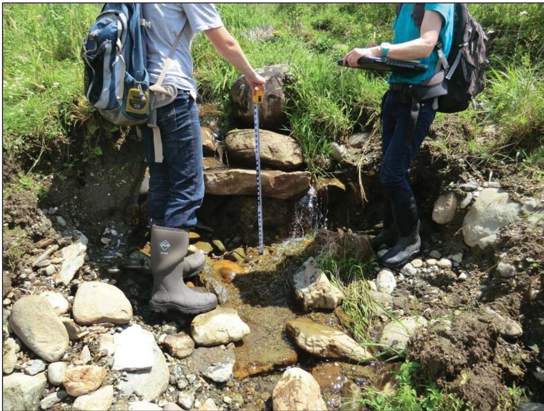
Figure 5.29. Headcut in M06S1.03.
