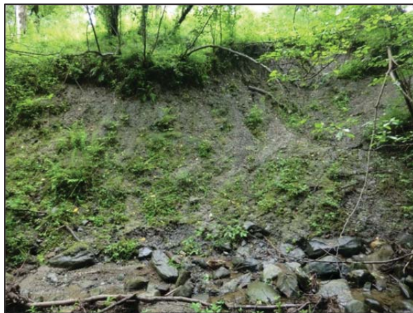
Figure 5.24. Photo of extensive mass failure along north bank in M04S1.02-C.
