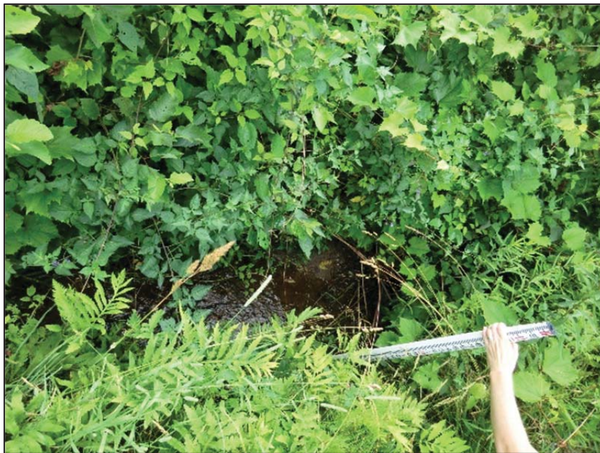
Figure 5.22. Photo of channel in M04S1.02-A.
