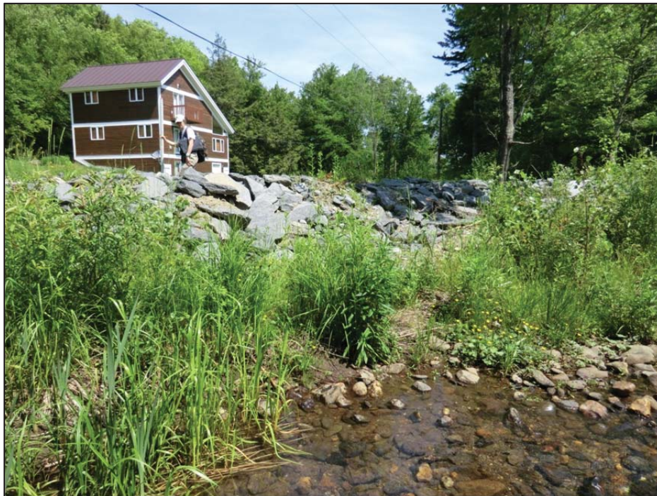
Figure 5.20. Large, recently constructed berm in T1.02-B.
