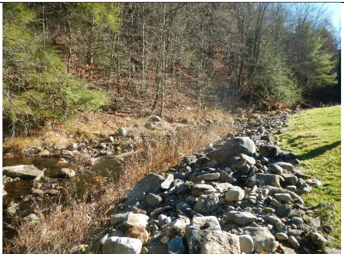
Bank straightening and armoring along cow pasture.
