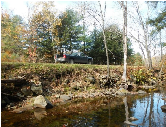
Figure 4.12: Bank erosion and failing armoring along Route 112 on reach M05.
