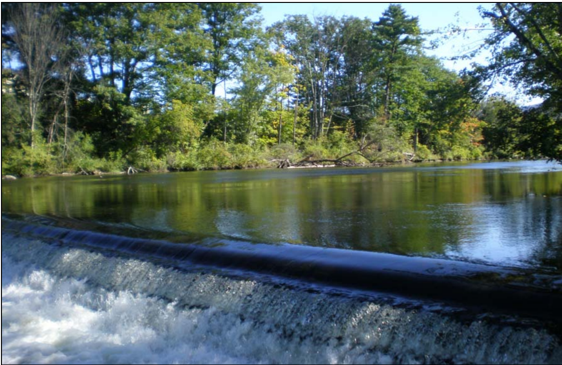
Figure 12. A small concrete dam, Ripley's Mills impedes sediment transport and alters flow at the upstream end of reach M21.
