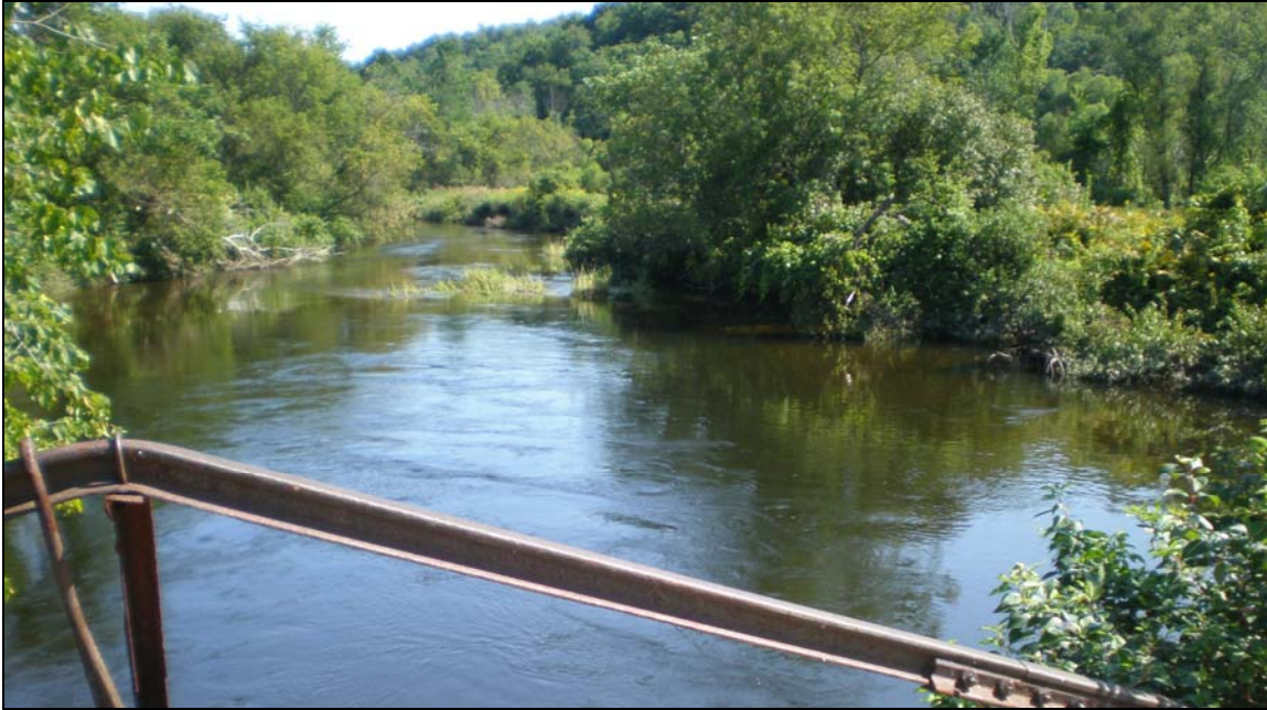
Figure 6. The view of reach M29 from one of several undersized crossing structures. Note the very wide, deep pool that has been scoured just downstream of this structure.
