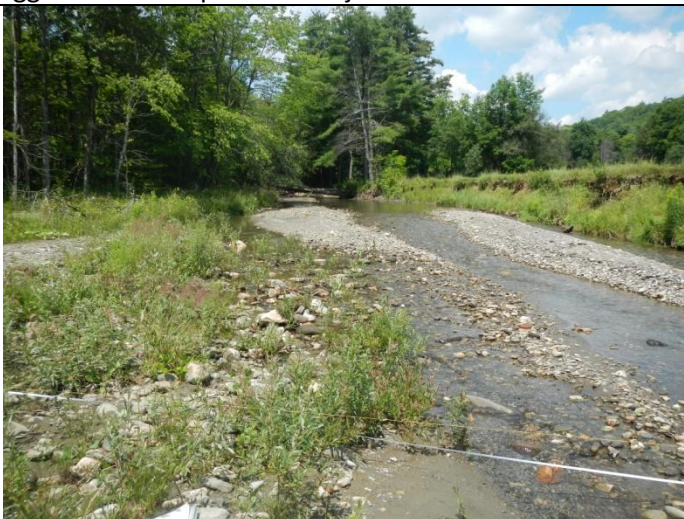
Widening and major deposition at the cross-section
