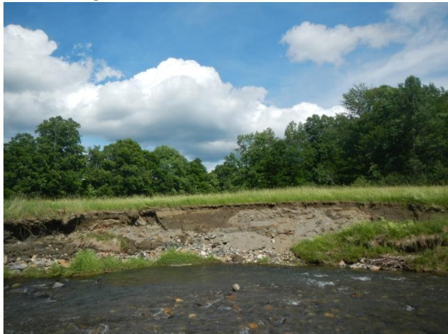
Figure 4.12: Major bank erosion and buffer impacts in reach M06.
