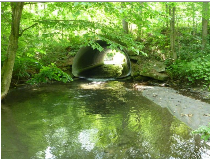
Coon Club Road culvert
