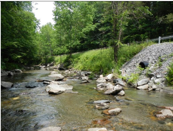
Encroachment and armoring along Rt 44
