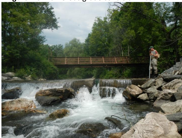
Figure 4.8: Small concrete block dam in reach M06.
