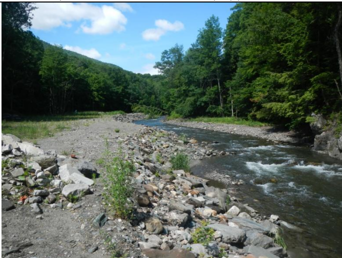
Channel and floodplain reconstructed in lower segment
