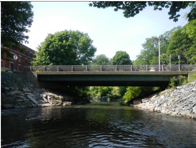
Bridge and armoring in the lower reach
