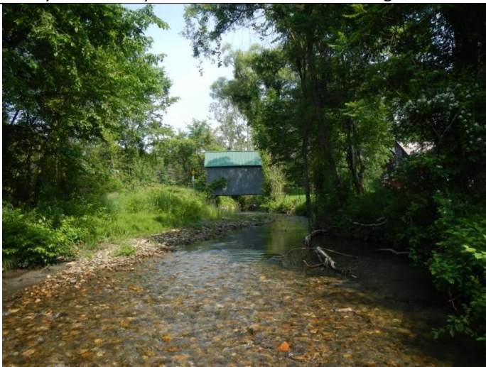
Churchill Rd bridge and accessible floodplain bench
