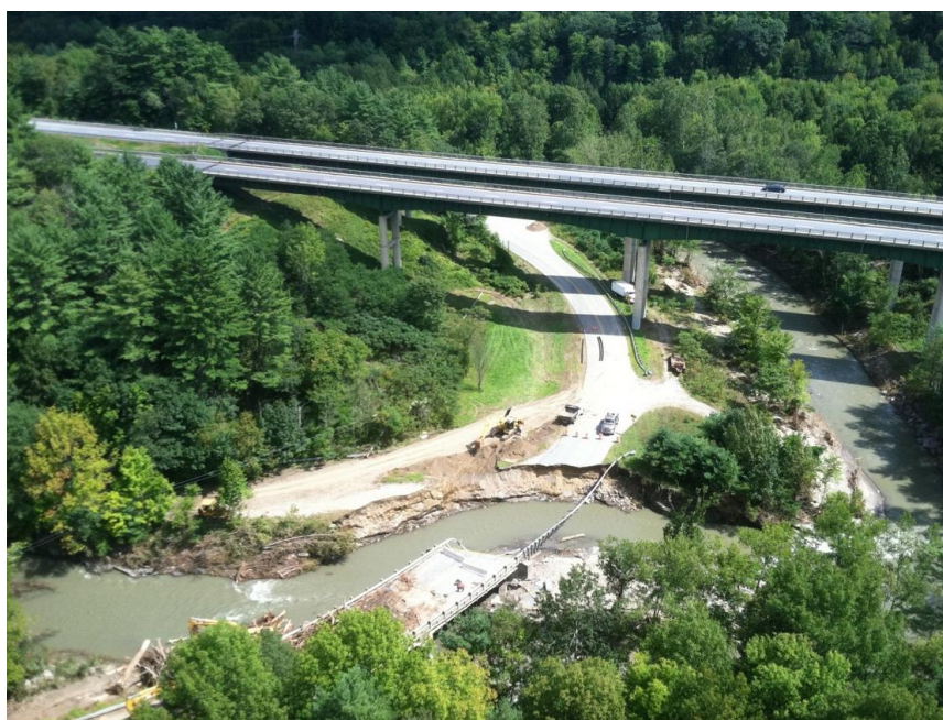
Figure 1.9: Route 44 bridge approach destroyed in Reach M04.
