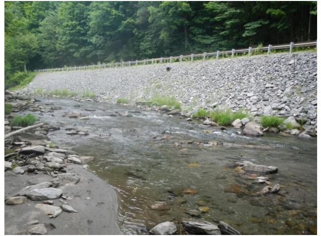
Figure 4.11: Harrington Road bank armoring in segment M07.B.
