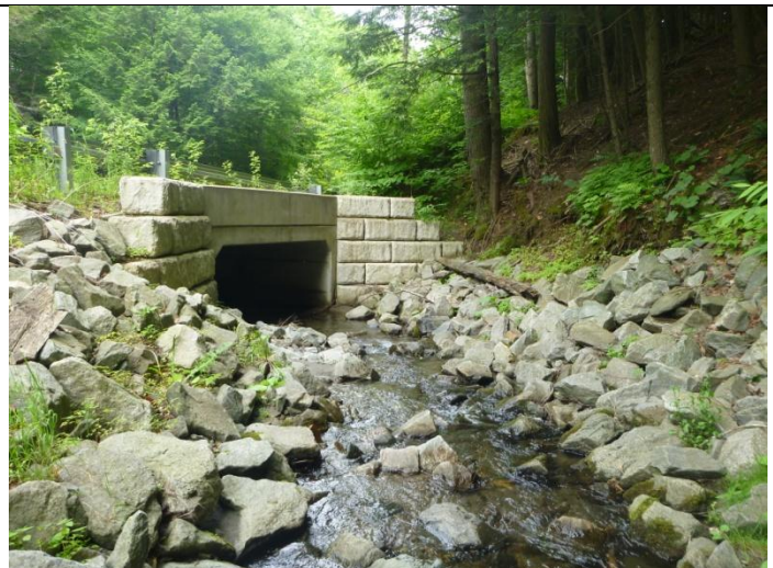
New box culvert under Sheddsville Rd
