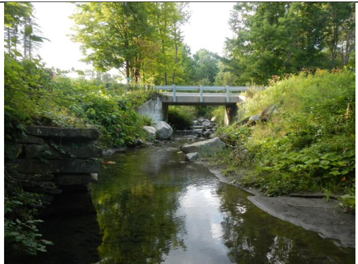
Several bridges and other constrictions increased incision
