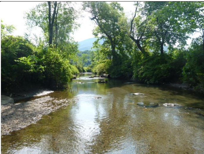
Deeply entrenched and incised segment
