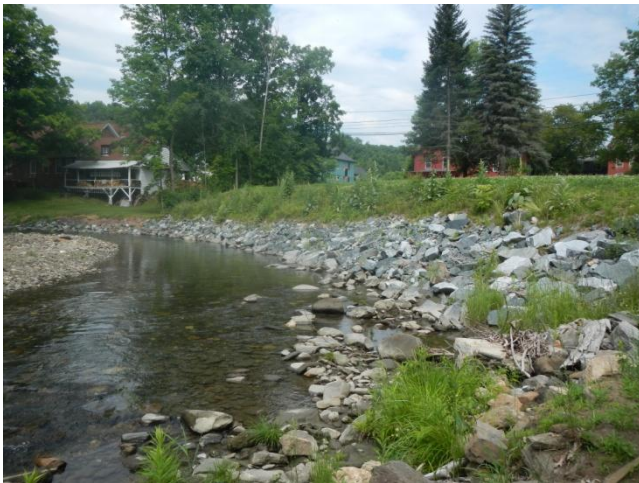
Figure 4.19: Encroachment from development in Brownsville on segment M07.A.
