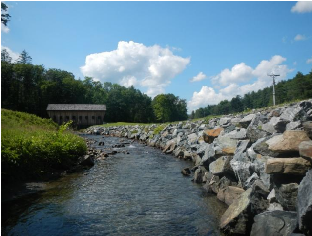
Figure 4.17: Recently straightened channel along reach M13.
