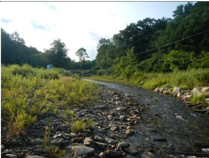
Straightening and encroachment along Bailey's Mills Rd
