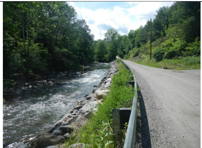
Accessible forested right floodplain and armoring along Brook Rd on left bank
