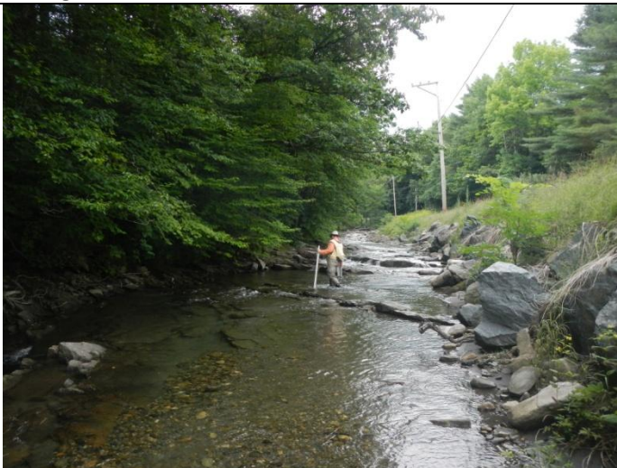
Incision and encroachment along Rt 106
