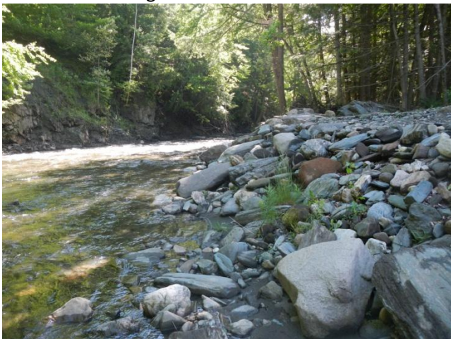
Figure 4.21: Dredged material blocking off a flood chute entrance on segment M05.B.
