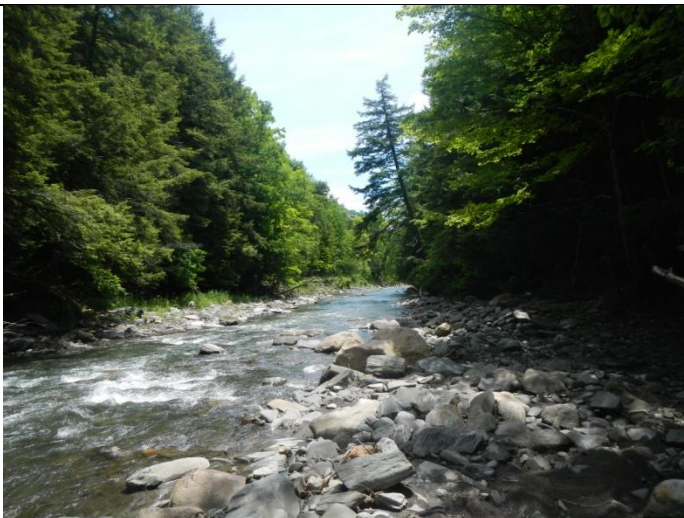
Minor scour and widening in lower segment, some floodplain access
