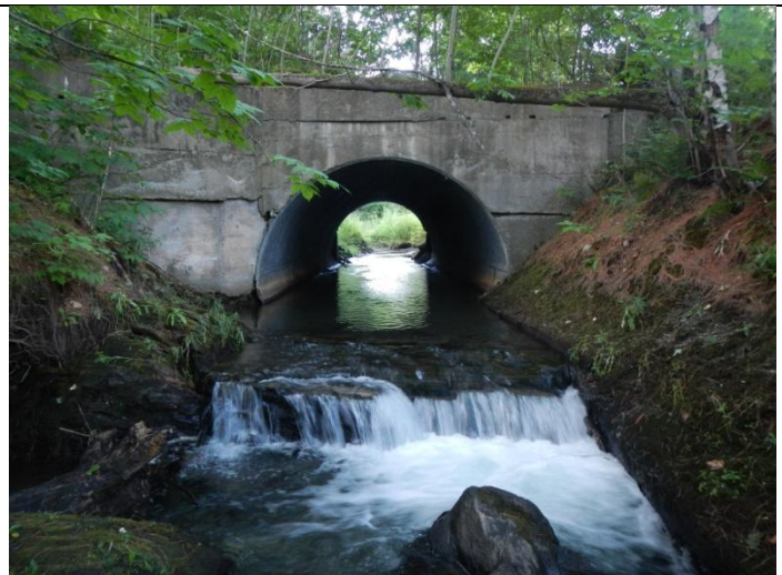
Ledge and mine access culvert
