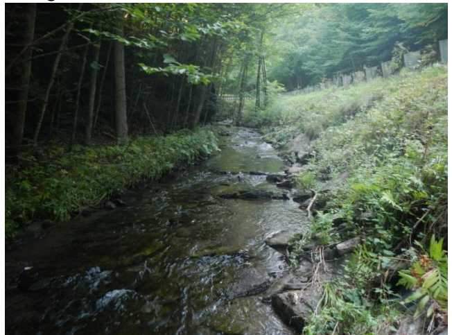
Figure 4.20: Extreme encroachment along Route 106 on reach T3.04.
