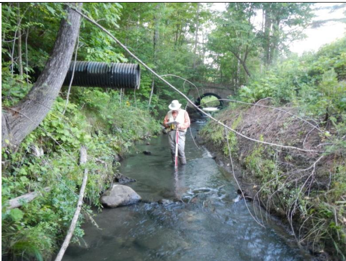
Straightened channel with ledge along right bank and poured concrete along left bank
