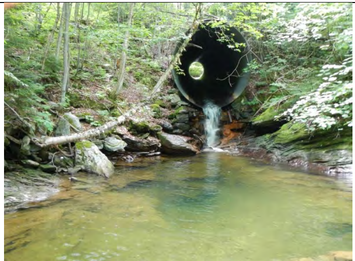
Large culvert under 108
