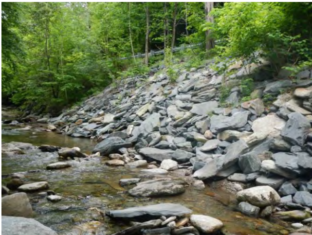
Figure 14: Encroachment from Desjardins Rd on T7.01.
