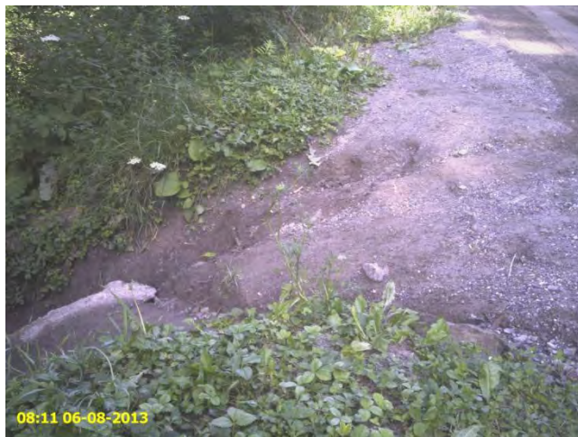
Figure 23: Entrance to Brewster River Trail from Canyon Road (photo by LCPC)
