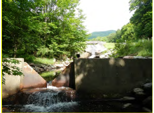
Figure 7: Weir and large dam on reach M14.
