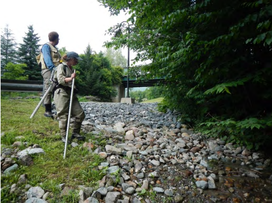
Figure 18: Roadside ditch conveying stormwater and sediment from West Hill Drive to reach T7S1.02.
