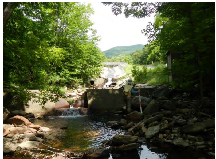
Large dam at the top of reach
