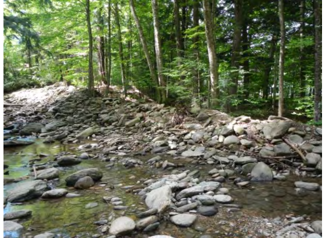
Figure 13: Recently constructed cobble berm blocking access to the left floodplain along reach M13.
