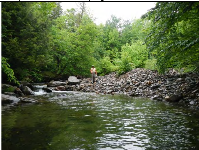
Major deposition upstream of Edwards Rd bridge
