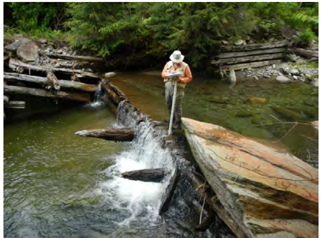
Figure 15: Partially breached timber crib dam on T7.01.
