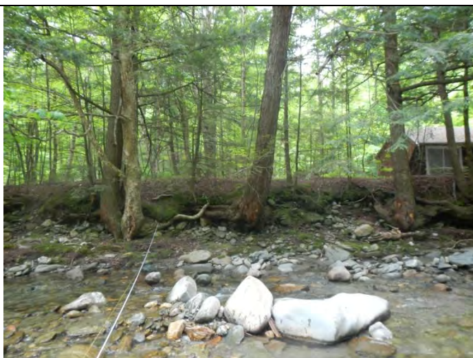
Recent bank scour along the campground property
