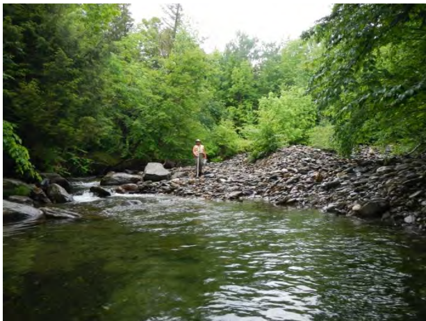
Figure 7: Huge cobble bar immediately upstream of the bridge
