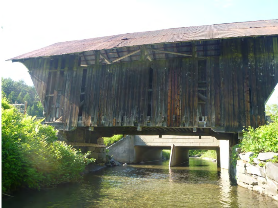
Figure 13: Covered bridge and box culverts on T5.02
