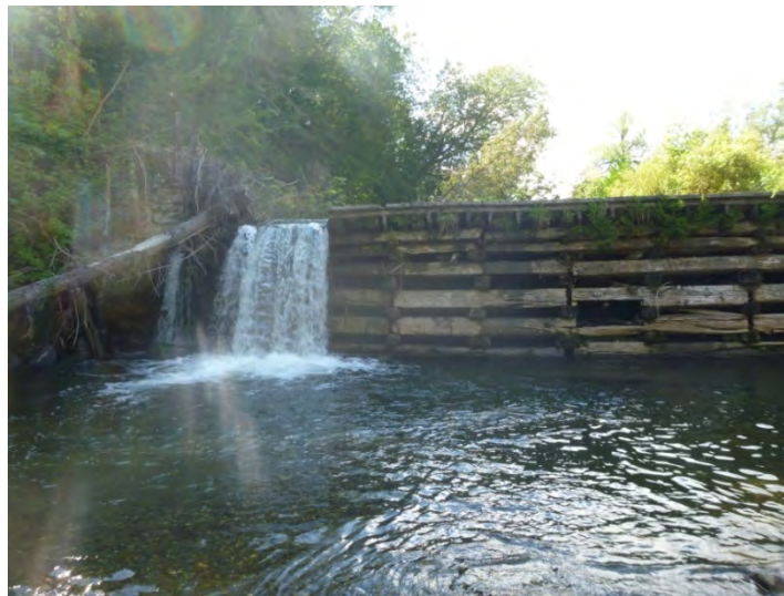
Figure 12: Timber crib dam on T3.10
