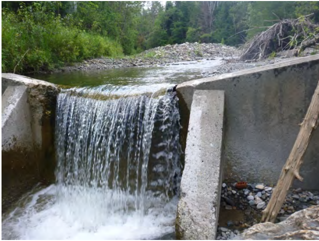
Figure 18: Sediment deposition upstream of abandoned USGS weir on T3.10S1.02
