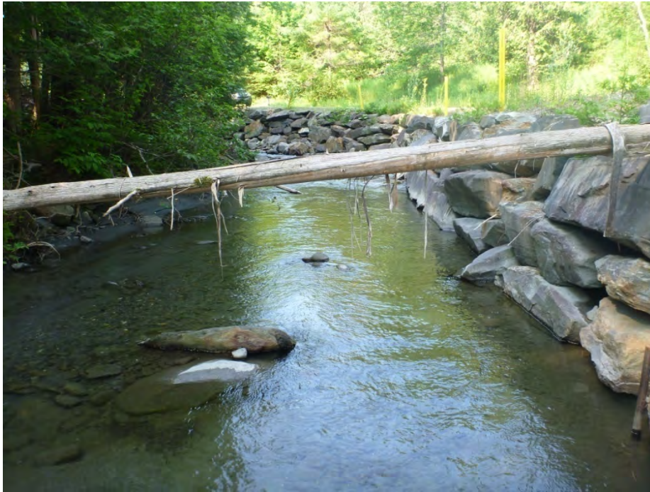
Figure 14: Bank armoring along Roy Rd in Reach T3.7S1.02
