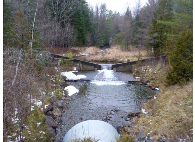
Figure 9: Active USGS weir in T3.14
