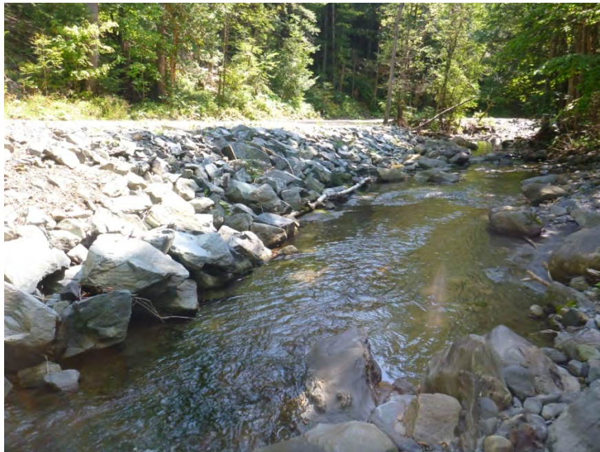
Figure 15: Encroachment from Water Andric Road along much of T2.08
