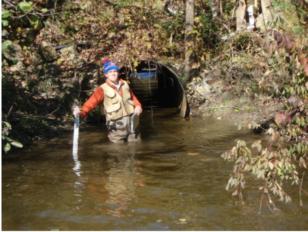
Figure 5.28 Scour pool downstream of the undersized culvert
