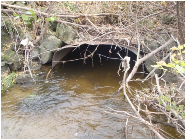
Figure 5.36 Downstream view of Sweeny Farm Rd culvert inlet
