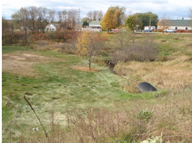
Figure 5.39 Downstream view from atop Allen Bk Drive culvert
