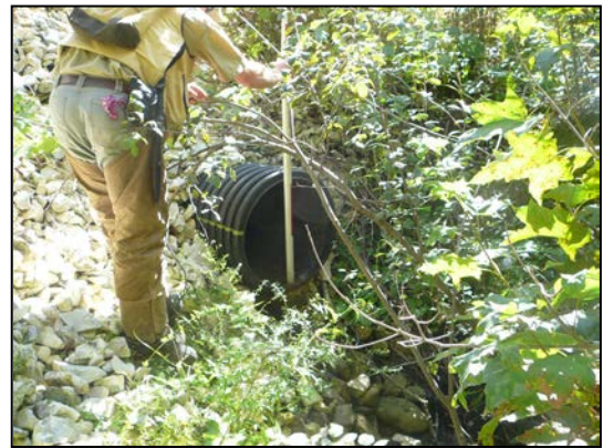
Figure 29. North Orwell Road culvert
