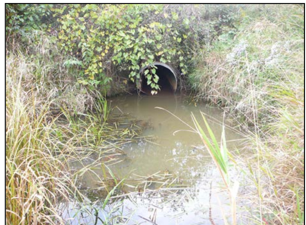
Figure 32. Outlet of Old Stage Road culvert
