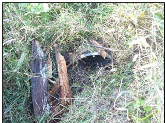
Figure 27. Upstream invert of farm road culvert
