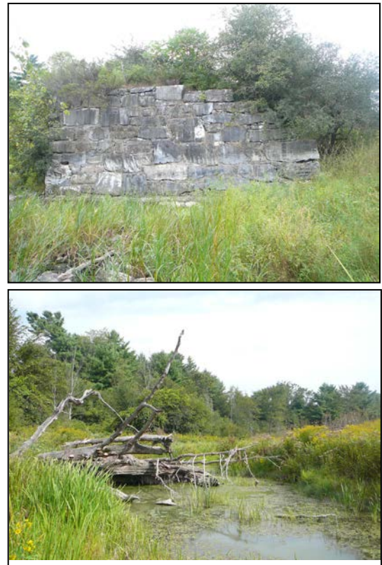
Figure 14. Old abutment on right bank and partial debris jam
