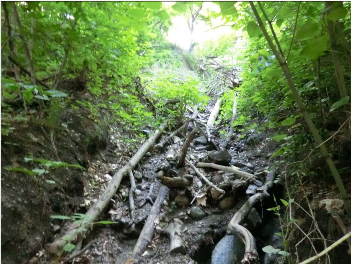
Figure 6.1. Gully erosion on west valley wall east of Lincoln Street (Project #1).
