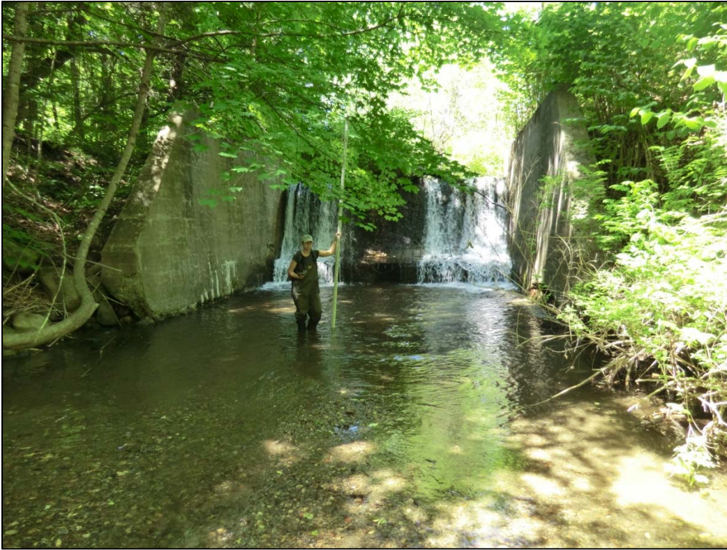
Figure 6.10. Old dam made of concrete that is 10.6 feet high.
