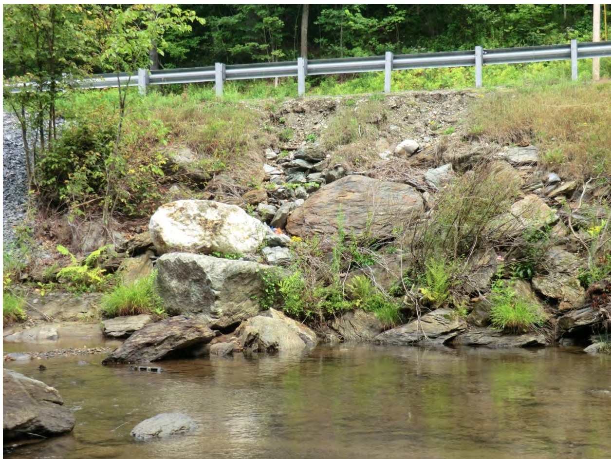
Figure 5.36. Storm water runoff from Route 4 on the northern bank.
