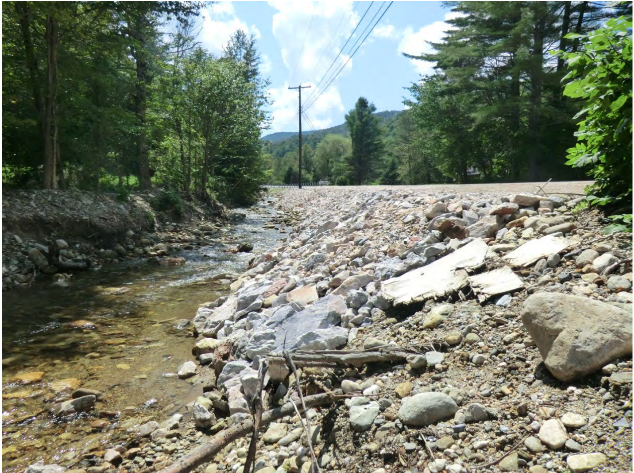
Figure 5.55. Channel straightening along Route 100 in M28T5.01-C.
