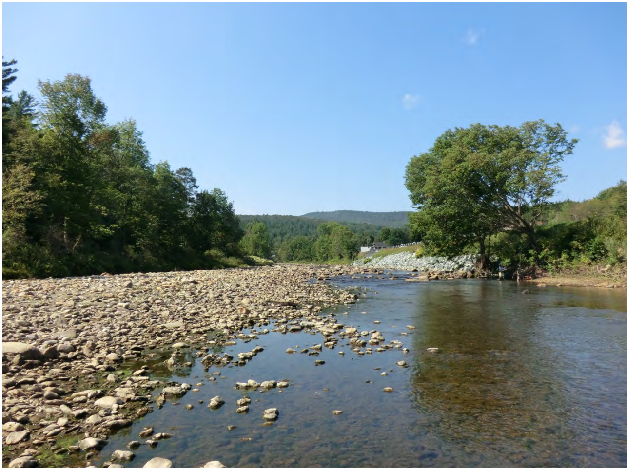
Figure 5.20. Typical channel in M21-D looking upstream. High aggradation. Lack of adequate buffer along Route 4.
