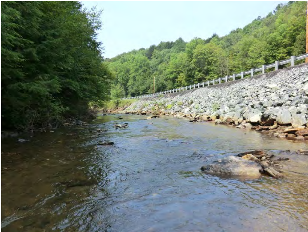
Figure 5.38. Typical channel for segments M27-A, M27-C, and M27-E. (Photo from M27-E.)
