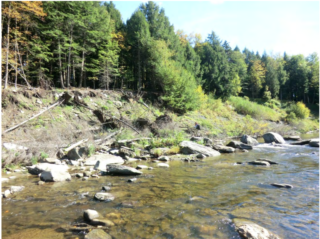
Figure 5.11. Mass failure on the southern bank at downstream end of M17.
