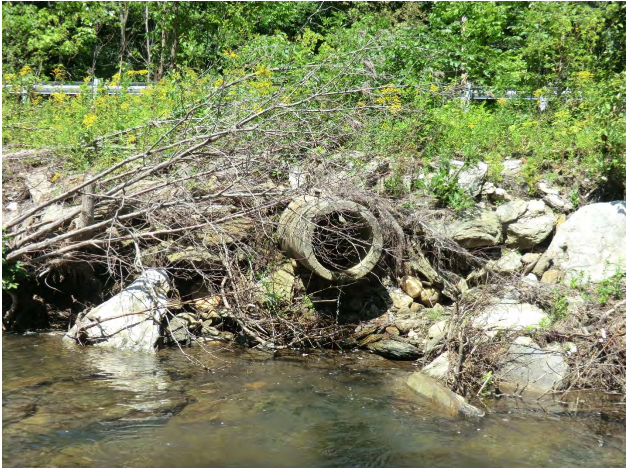
Figure 5.44. Storm water input along Route 4 in M28-A.
