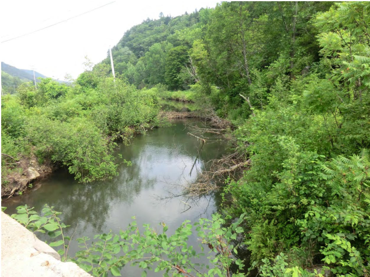
Figure 5.52. Beaver dam upstream of Route 4 bridge crossing.
