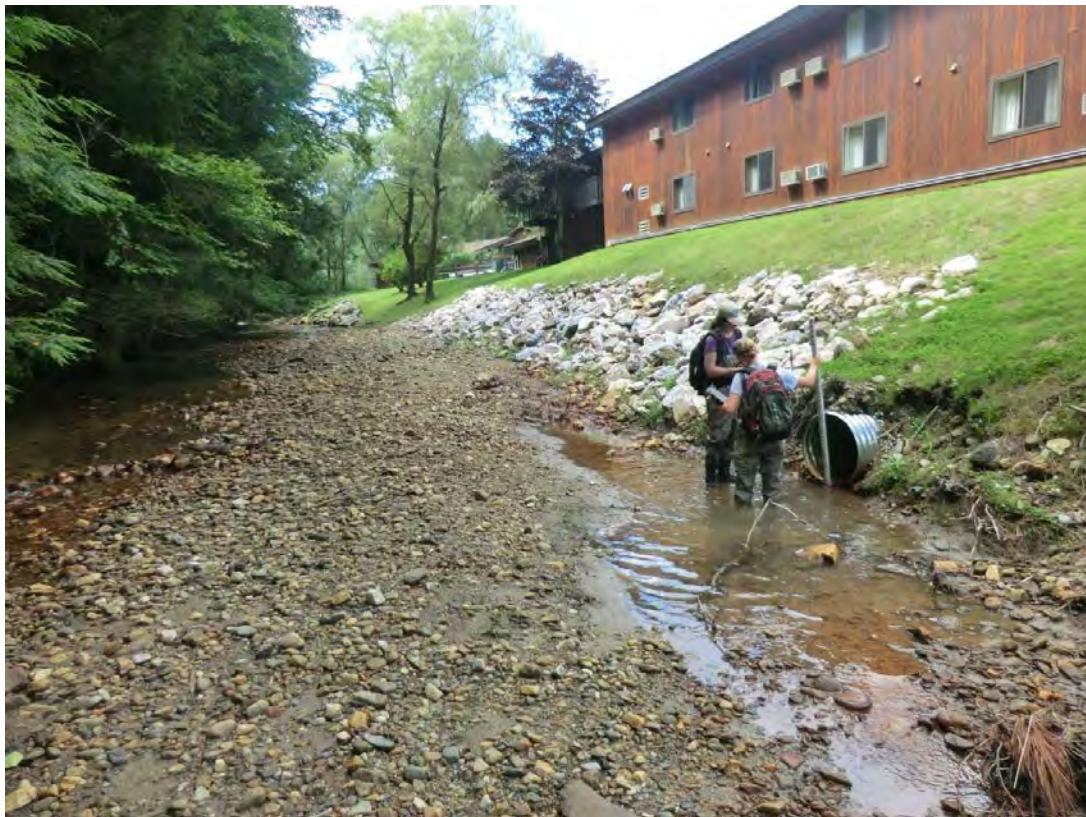
Figure 5.53. Stormwater input in M28T5.01-A. Major aggradation, poor buffer, and riprap are seen here.
