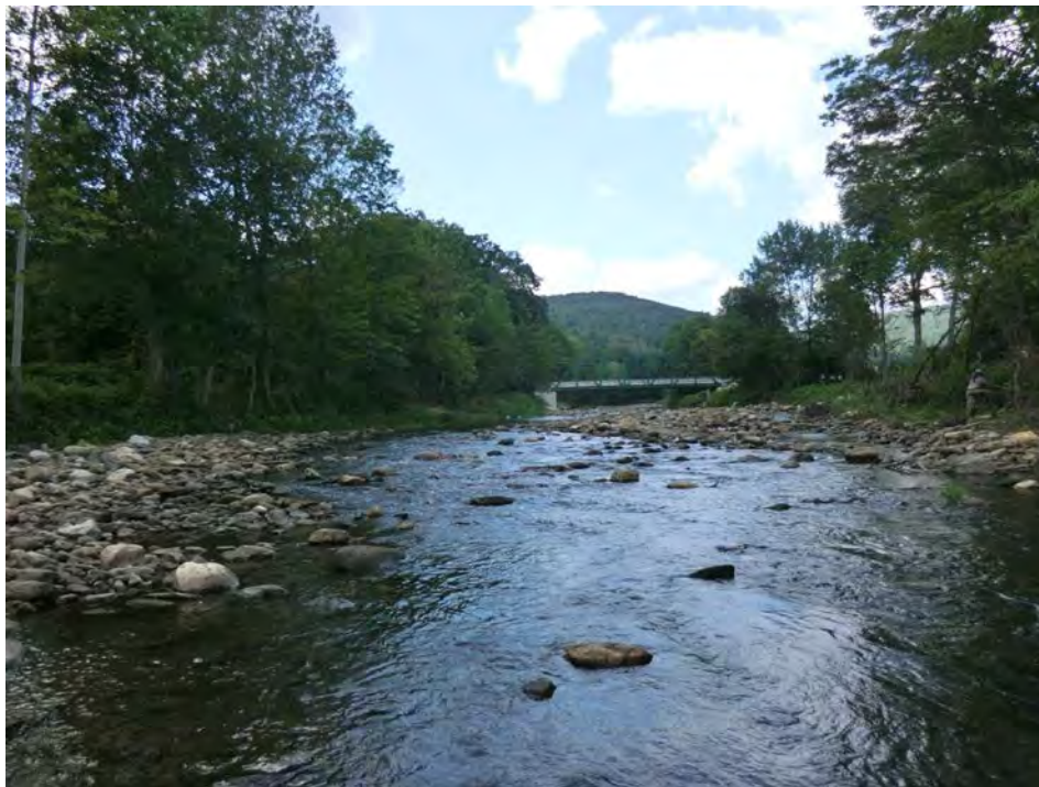
Figure 5.27. Typical channel in M24-A includes major aggradation. Route 100A bridge is upstream.
