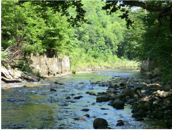
Project #4 – Investigate Abutment Removal
