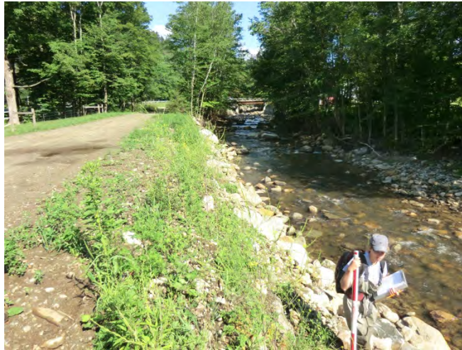
Project #6 – Create Floodplain/Streamside Plantings
