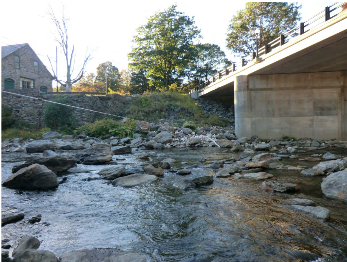
Figure 5.9. Extensive channel straightening seen through rip rap and hard bank armoring.
