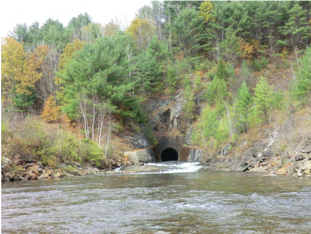
Figure 5.10. Outflow of the Union Village Dam.
