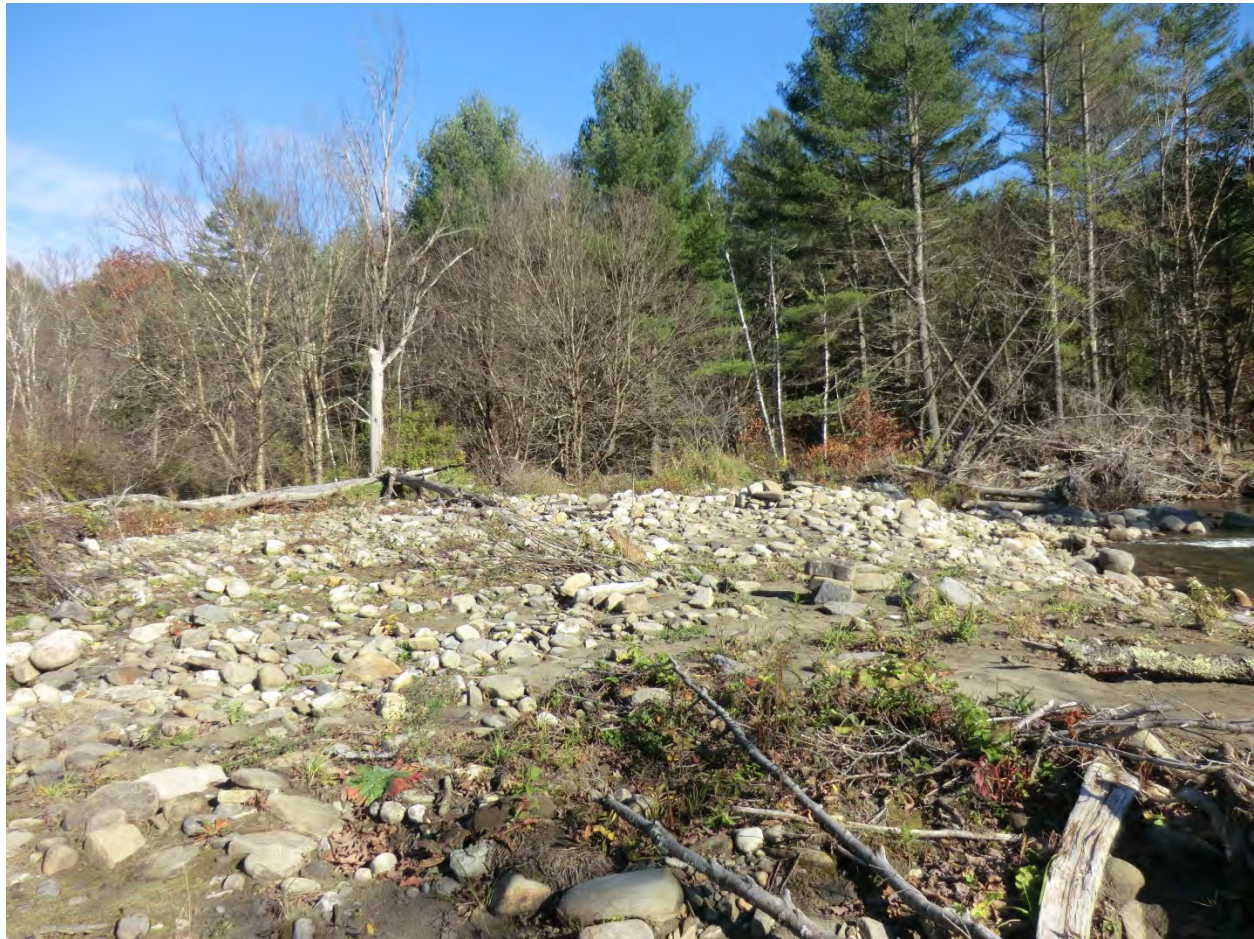
Figure 5.41. A channel avulsion has created this island in M01-E. Major aggradation can be seen here as well.
