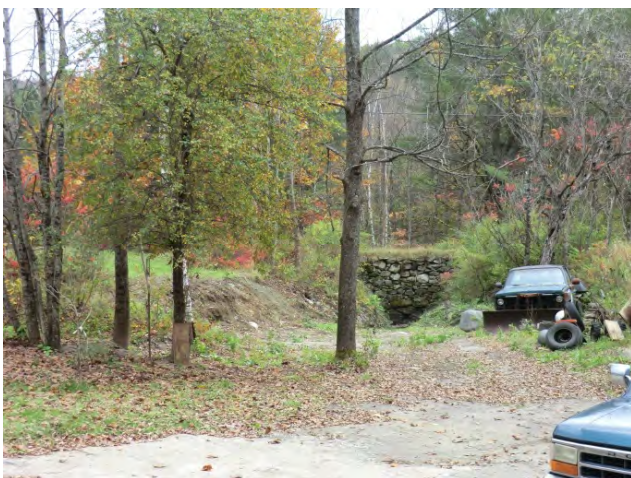
Project #2 – Old Abutment Removal, M02
