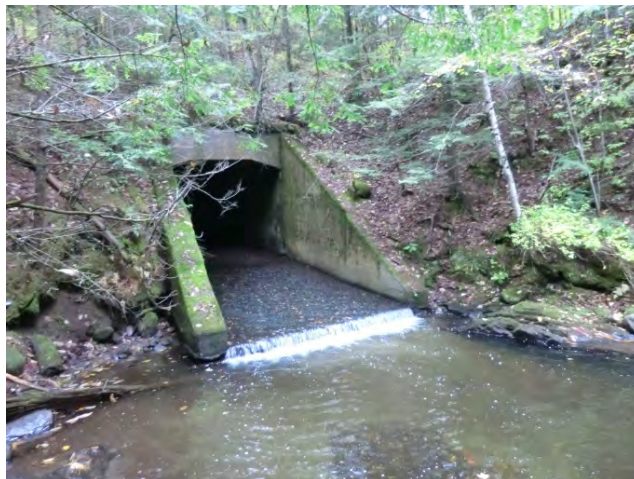
Project #4 – Replace Box Culvert, R06.S1.02-B
