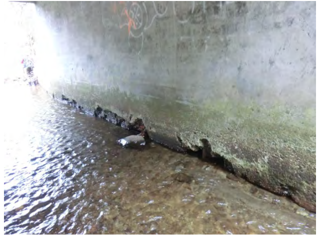
Project #1 – Replace Box Culvert R06.S1.01-B
