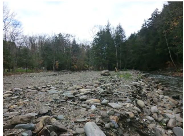
Project #3 – Restore Natural Channel, M02
