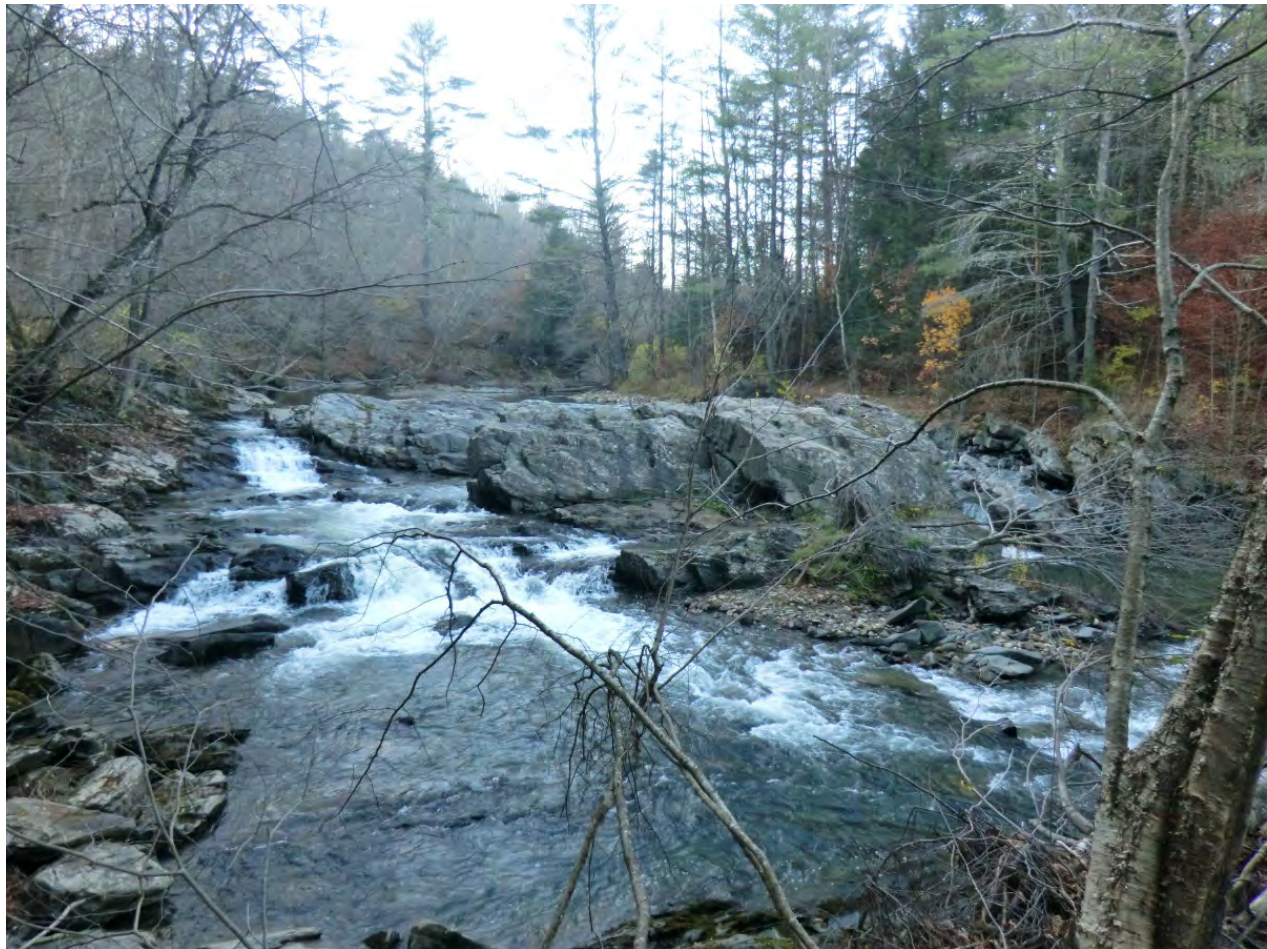
Figure 5.37. Downstream end of M01-B is a large bedrock grade control.
