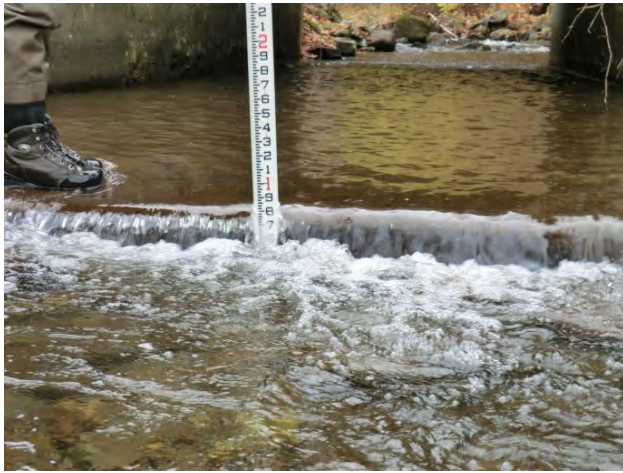
Project #1 – Replace Box Culvert, R06.S1.01-B
