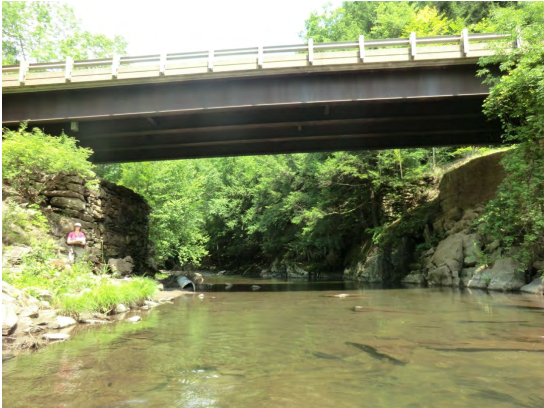
Figure 5.29. Old bridge abutment beneath Sawnee Bean Road bridge is causing a channel constriction.
