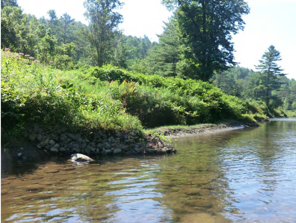
Figure 5.14. Gabions at the stream edge in segment R08-B likely contributed to historical channel straightening.
