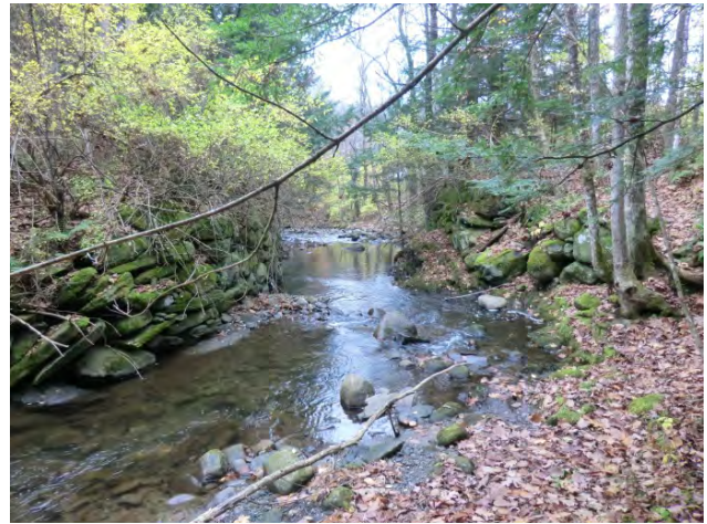
Project #3 – Remove Old Abutment R06.S1.01-B
