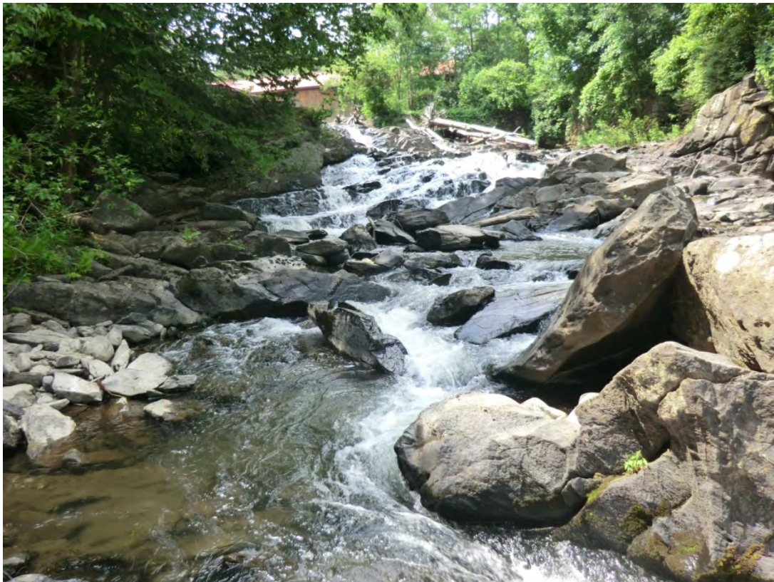
Figure 5.22. Looking upstream at a section of grade controls in R10-C.
