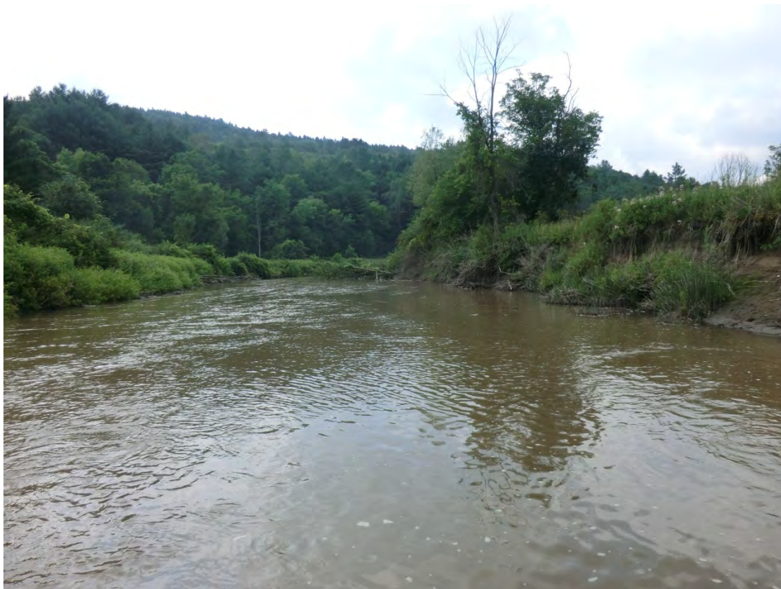
Figure 5.18. Typical eroded banks and limited bank and buffer vegetation in R09.
