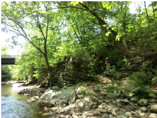
Project #5 – Remove Old Abutment, R12-A
