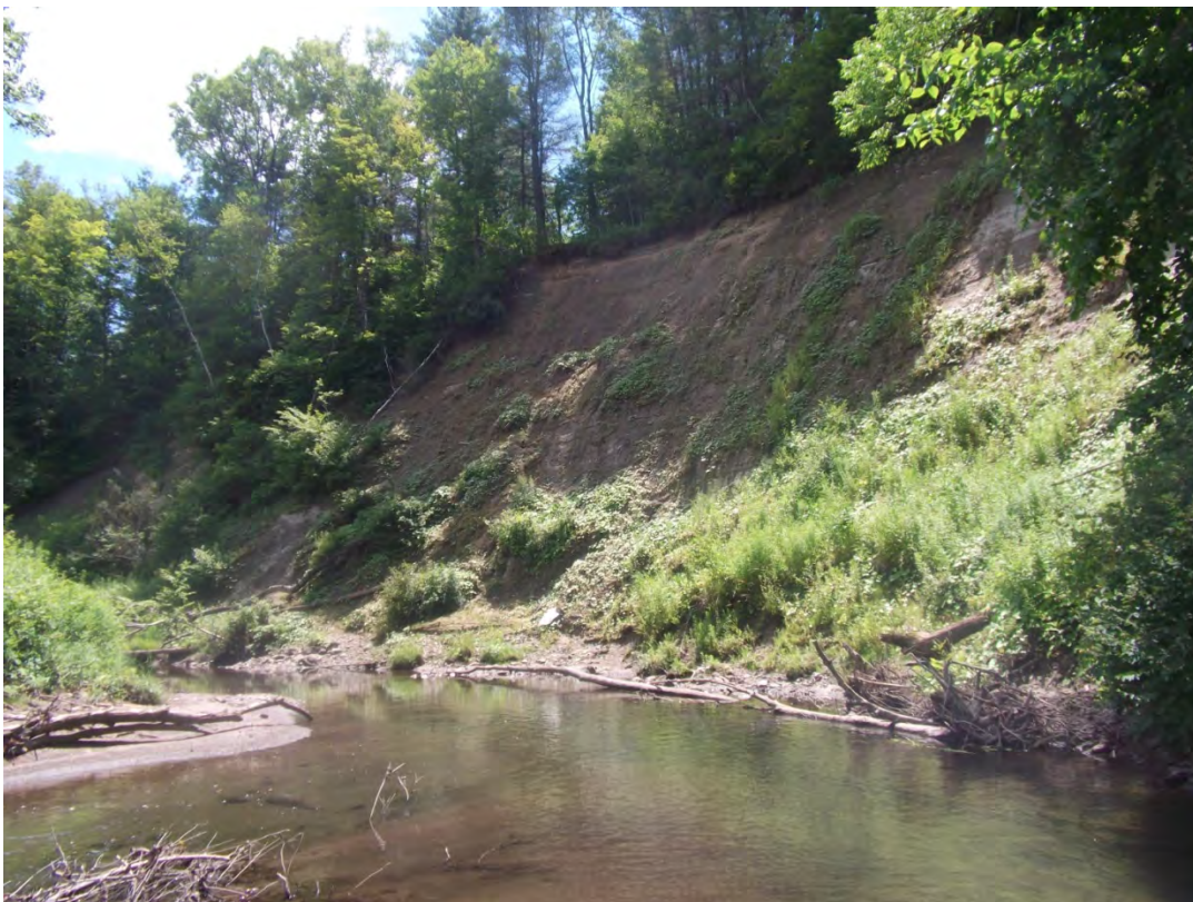
Figure 5.26. Large mass failure on the valley wall.
