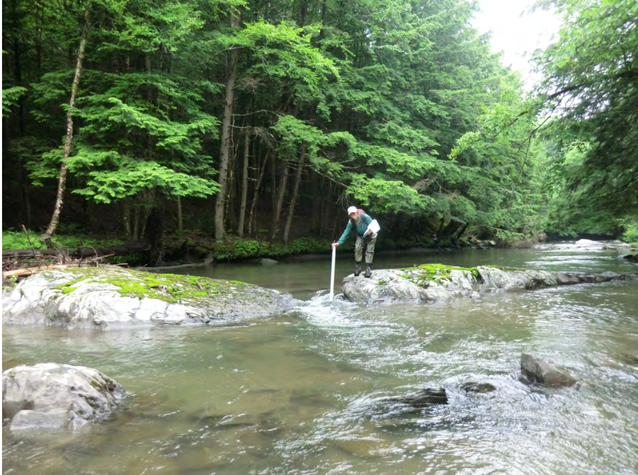
Figure 5.33. Bedrock grade controls in R14-A help to keep this segment in a stable geomorphic condition.
