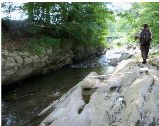
Figure 4.14 Ledge grade control above Geer dam
