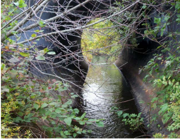
Project #7- Culvert Replacement
