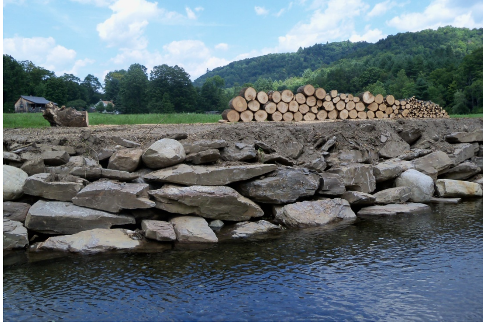
Figure 4.16 Newly installed riprap with trees cut along the bank in segment R19-B
