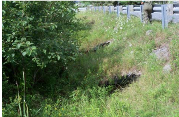
Figure 4.76. Three culverts at Route 244 Crossing
