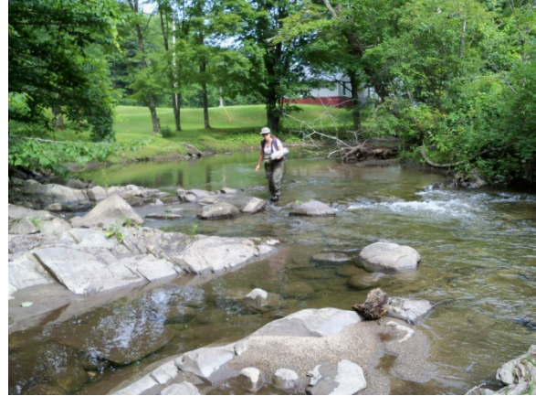
Figure 4.18 Ledge grade control in R20-A
