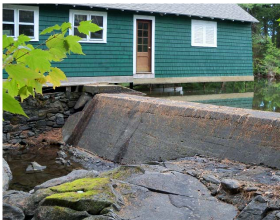
Figure 4.28 Lake Fairlee Dam from downstream
