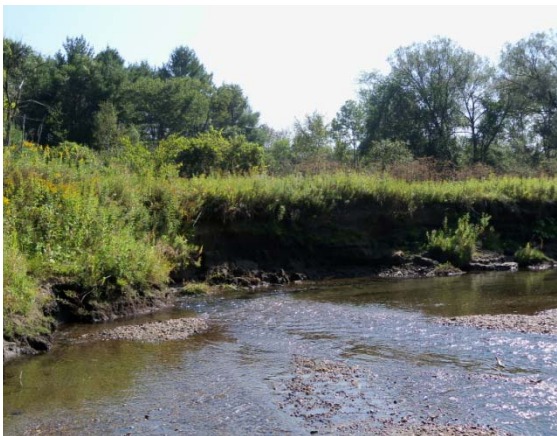
Figure 4.8 Extensive bank erosion in Reach R17
