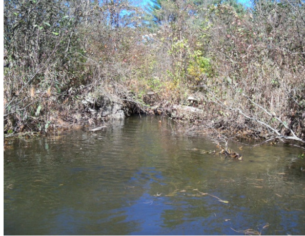
Project #2 – Remove old abutment
