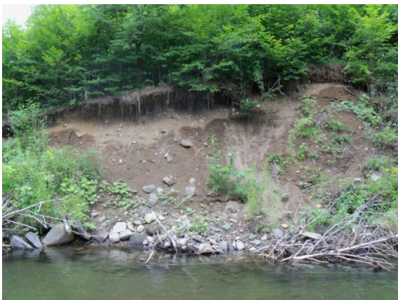
Figure 4.19 Mass failure on east bank
