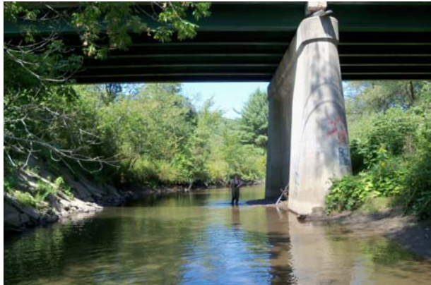
Figure 4.75. Center pier of Route 244 Bridge
