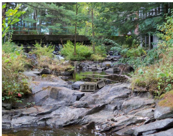
Figure 4.29 Looking upstream at natural ledge & Dam
