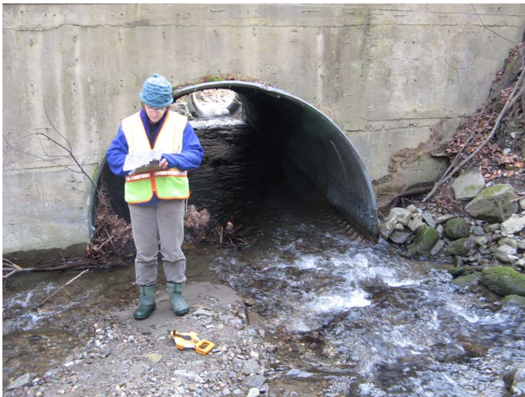
Figure 5 – Double culvert on Barker Brook, Thetford, with midchannel bar
