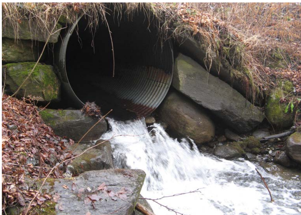
Figure 1– Perched Outlet on Vershire Center Road
