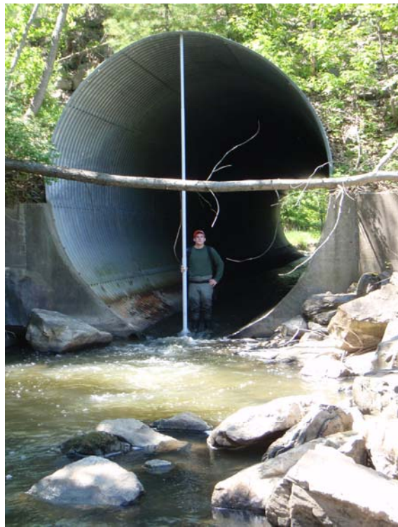
Figure 22. Culvert crossing at Marshall Ave.
