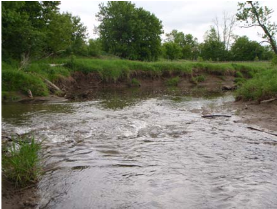
Figure 15. 0.5-foot head cut (picture taken upstream)
