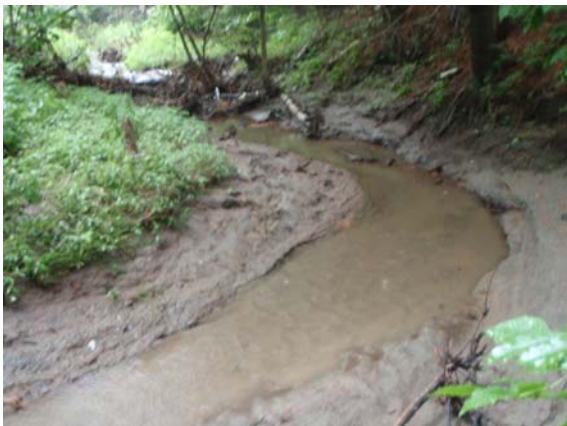
Figure 48. Aggradation of sediment mid-segment
