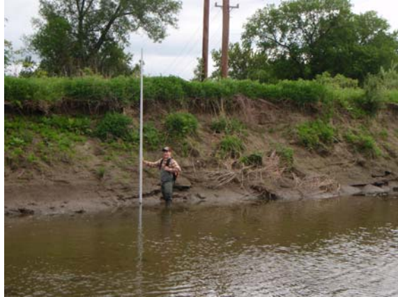
Figure 14. Bank erosion on the right bank 10'h x 150' l
