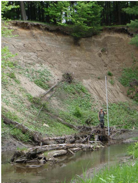
Figure 16. Mass failure on the right bank 40'h x 70'
