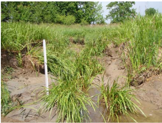
Figure 50. The gully created by the three headcuts
