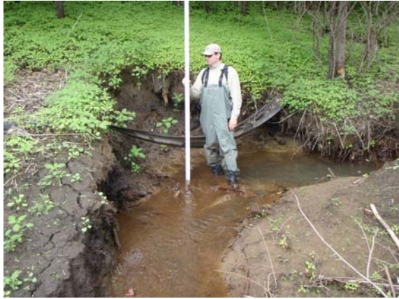
Figure 43 Bank erosion above Marshall Ave. crossing.
