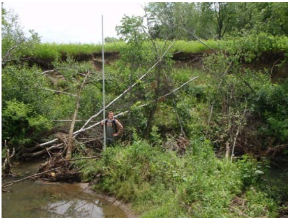
Figure 46. Mass failure on left bank (mid-segment)
