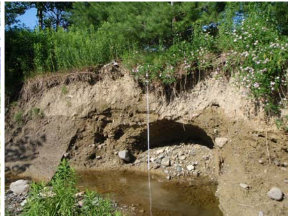
Figure 56. A mass failure observed on the left bank
