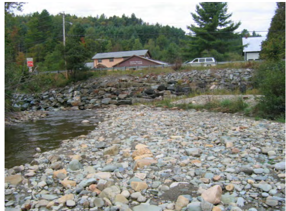
Figure 7.13. Rock riprap along North Wolcott Road in reach T09
