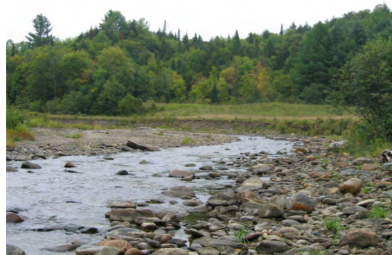
Figure 7.12. Bank failure on outside bend in reach T08 where the buffer is less than 25 feet in width.
