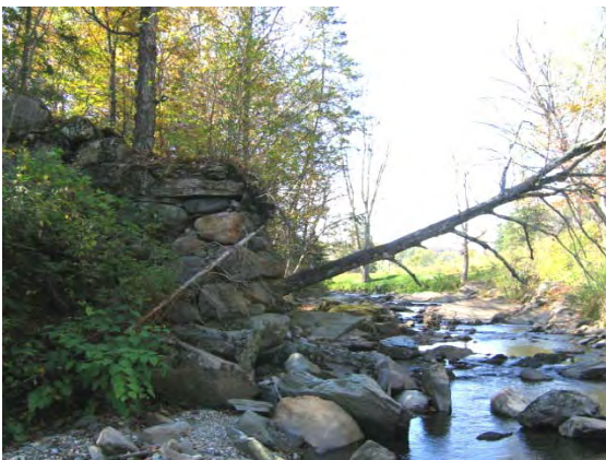
Figure 7.30. Remnants of possible historic dam in segment T15-C.
