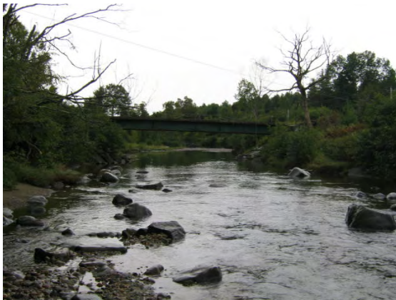
Figure 7.6. The Wild Branch Lane Bridge is a floodprone constriction and not a channel constriction.
