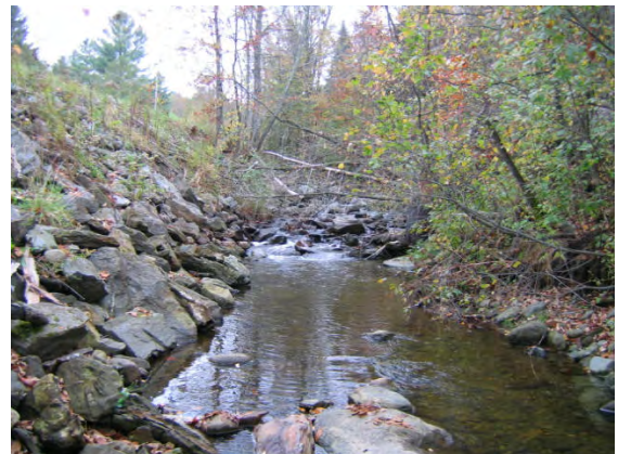
Figure 7.42. A steep riffle is shown upstream of the riprap that is located along Brook Road in Reach T10.01.
