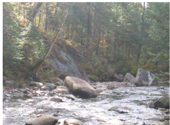
Figure 7.38. Erosion along the east bank. This bank contains clay.
