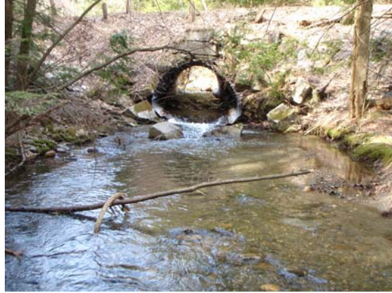
Figure 28. Houghton Road culvert in upper M06-B
