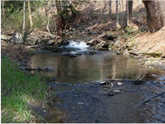
Figure 42. Old dam in lower T1.02-E.
