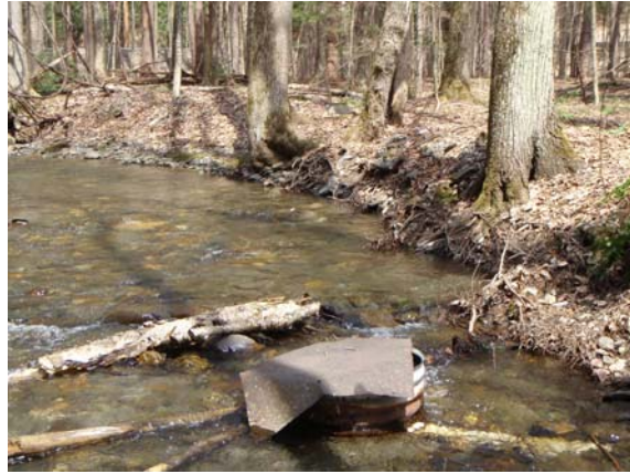
Figure 26. Cistern pond diversion in M06-A.
