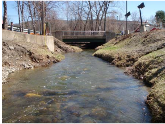
Figure 15. M01-B above Route 5 crossing.
