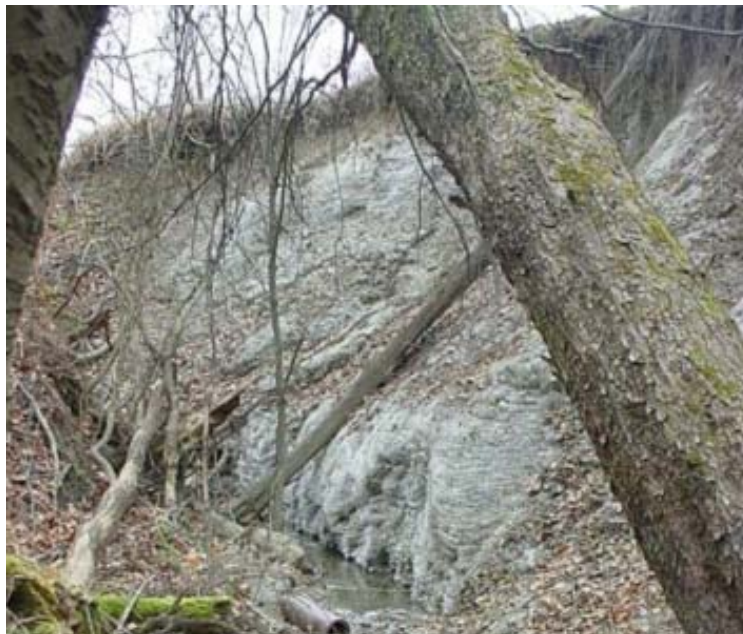
Figure 9. Gully on Pepsi Property draining to lower Reach M03.
