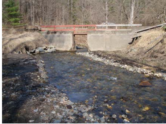
Figure 30. Dam and sluice gate in upper M06-C.
