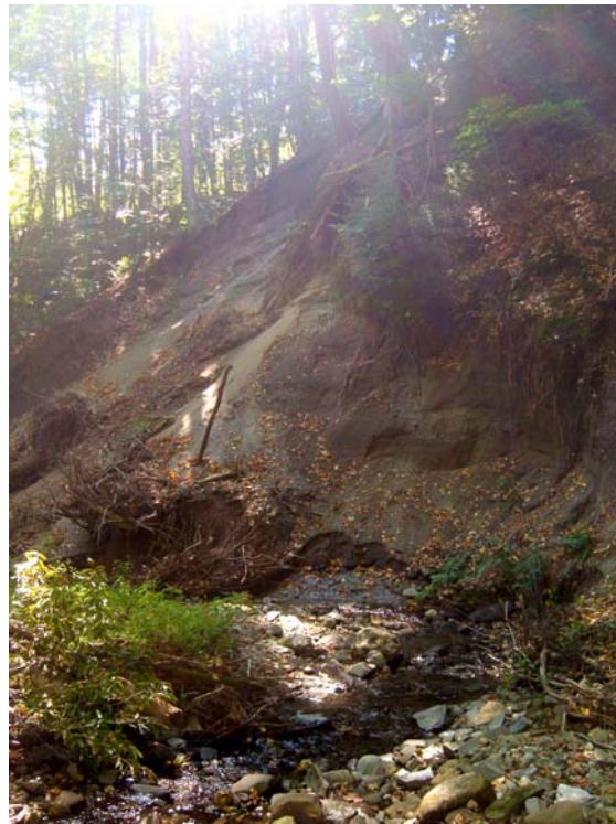
Figure 9. Large landslide in lower T1.02
