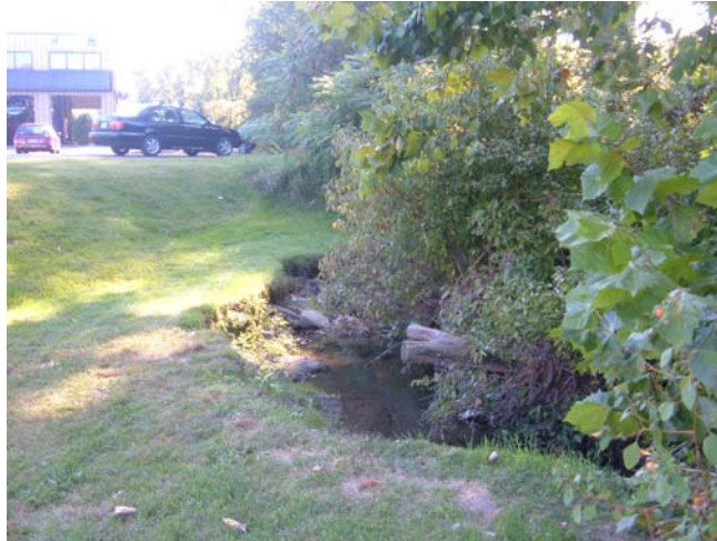
Figure 6. Bank erosion and lack of woody vegetative buffer in M02.
