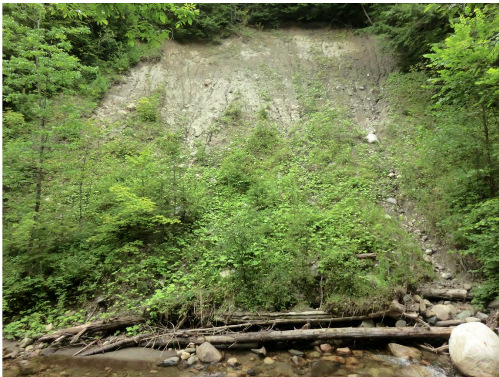
Figure 5.12. Mass failure on the northern bank in reach M103.
