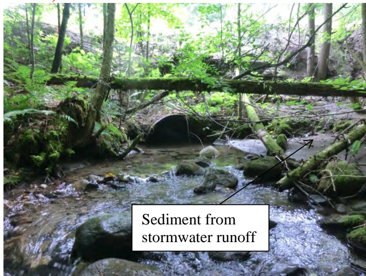
Stormwater runoff off of trail crossing by culvert in T1.02
