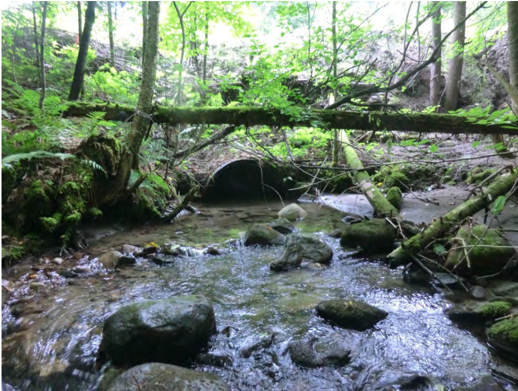
Figure 5.25. Stormwater input from trail just upstream of reach T1.01.
