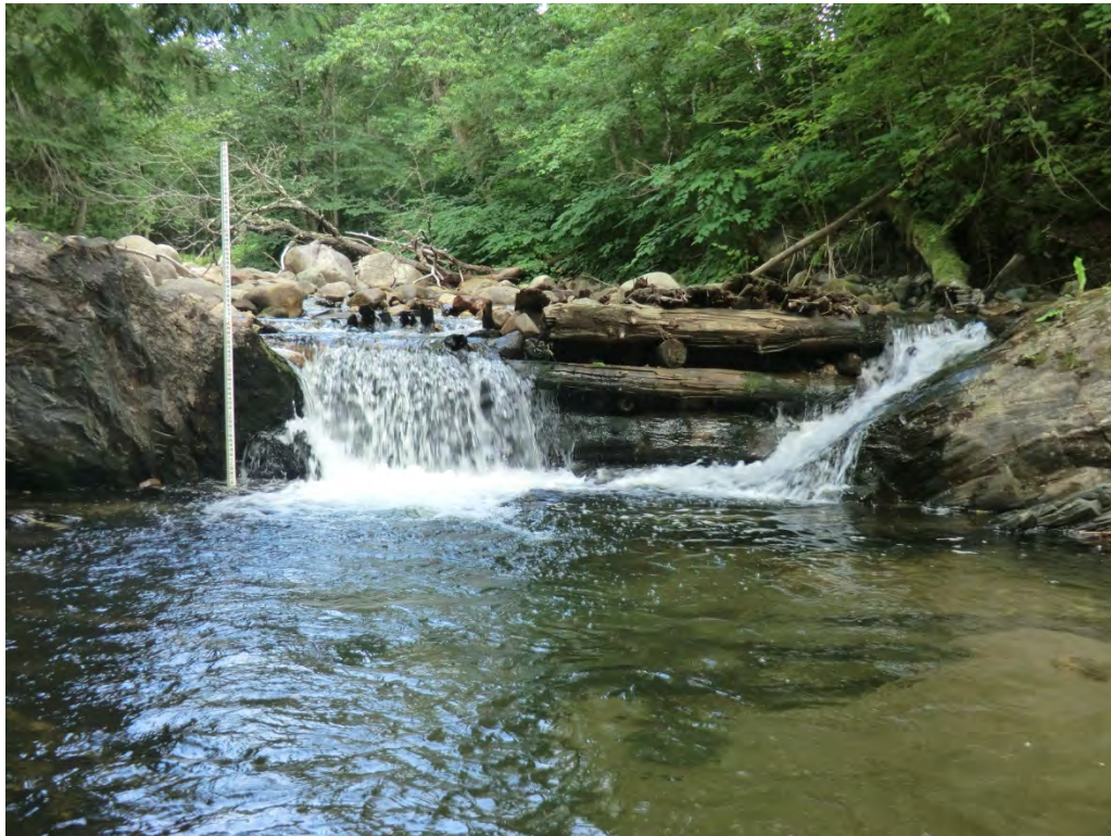
Figure 5.8. Old dam with logs in channel causing scour downstream in M102-A.
