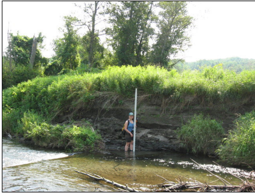
Figure 30: Eroding banks along reach M09
