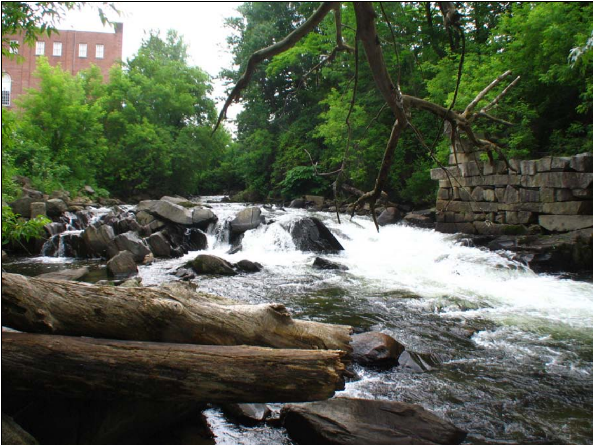
Figure 20: Bedrock ledge and old mill foundation along Reach M04A.
