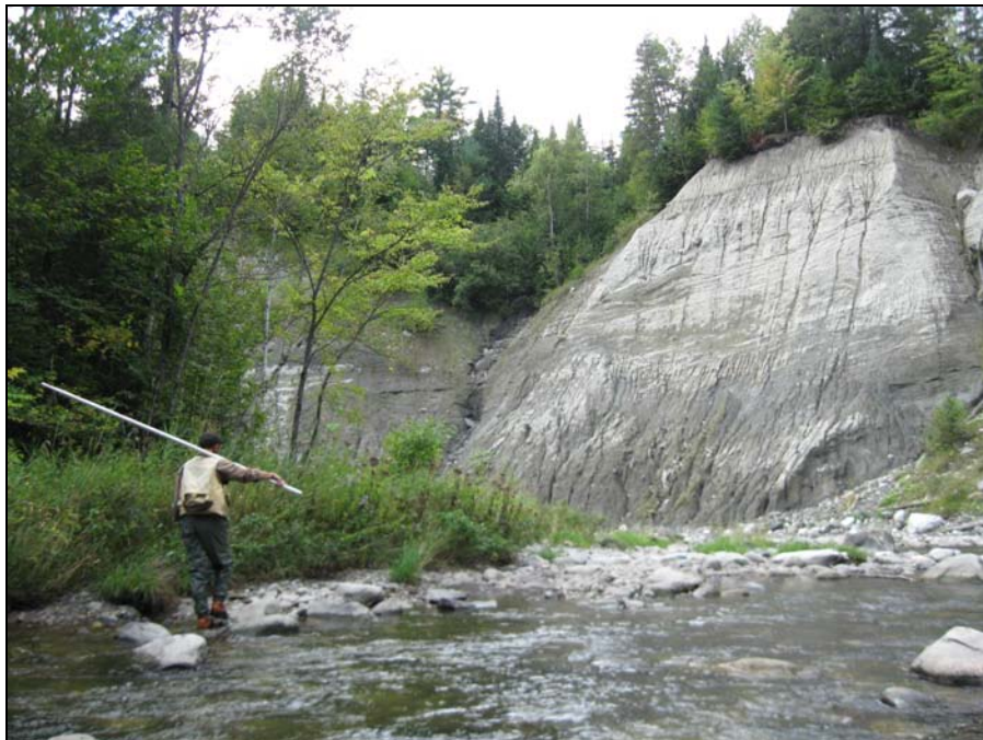
Figure 38: Typical section of the Willoughby River (Reach T3.03, above); One of several mass failure sites on the Willoughby River (Reach T3.04, below).
