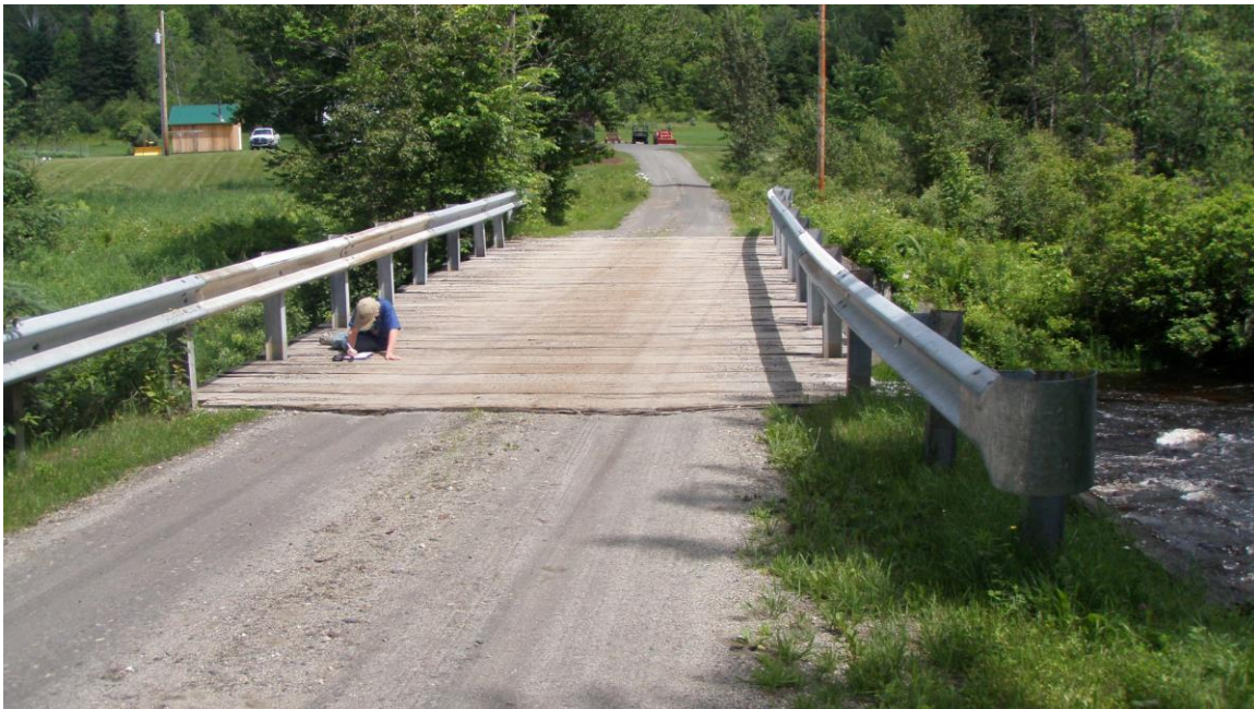
Photo 9. Fournier Bridge. Dividing Reaches M12B and M12A.
