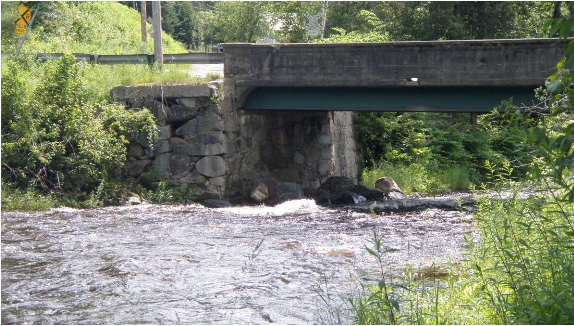
Photo 7. The bridge at the bottom of Reach M12A.
