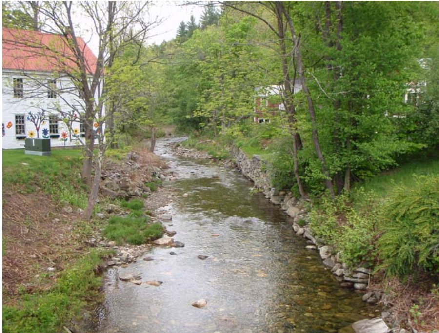
Figure 17. Corridor encroachment in Grafton Village in Reach M14.
