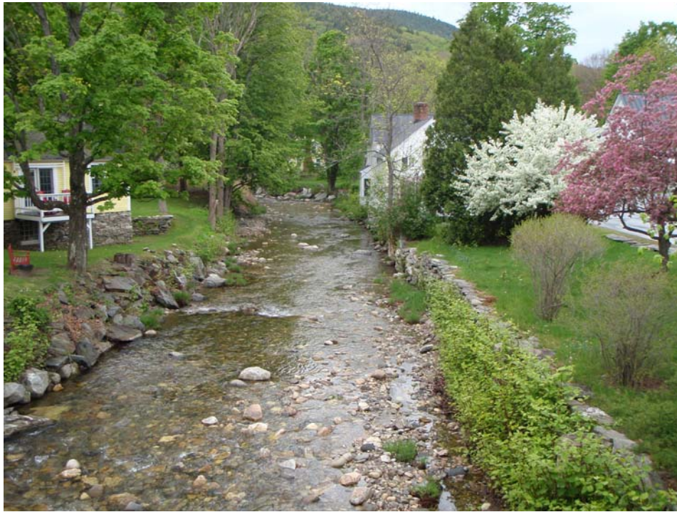
Figure 15. Hard bank armoring protecting adjacent properties in M14 in Grafton village.
