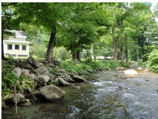
Figure 4.31 Rip-rap on the right bank downstream of Main St
