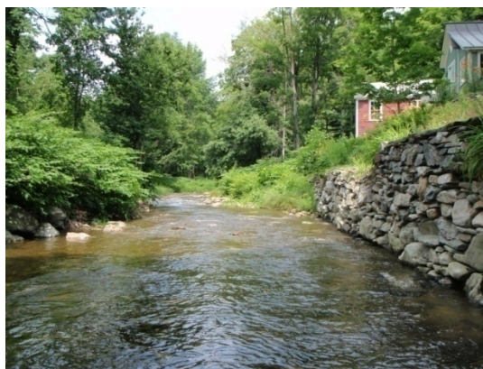
Figure 4.32 Hard bank upstream of the Main Street
