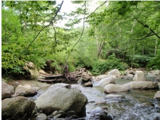
Figure 4.43 The left bank prior to rip-rapping
