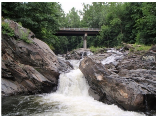
Figure 4.7 The grade control downstream of Covered Bridge Rd
