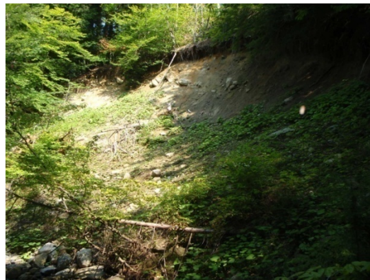
Figure 4.85 Mass failure on the left bank
