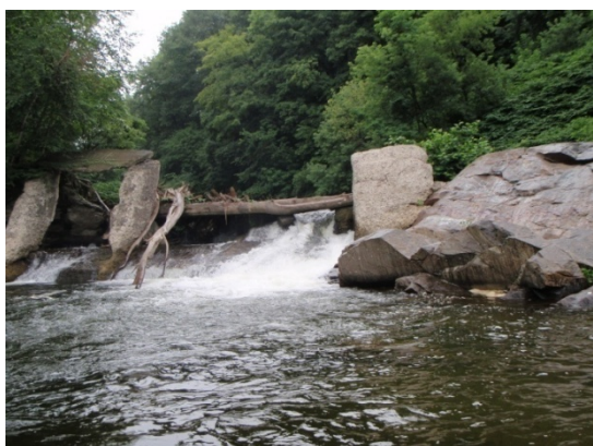
Figure 4.1 Blake and Higgins dam buttresses on a grade control
