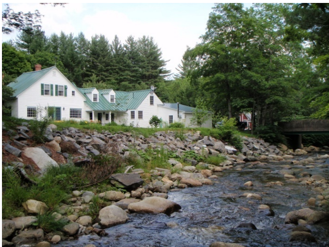
Figure 4.42 Armoring and no buffer upstream of the Cabell Road Crossing on the left bank
