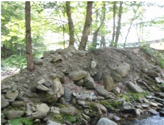
Figure 4.88 Dredging pilings on the right bank
