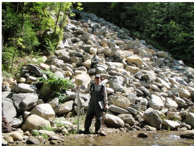
Figure 4.39 Mass failure on the right bank that has been heavily armored
