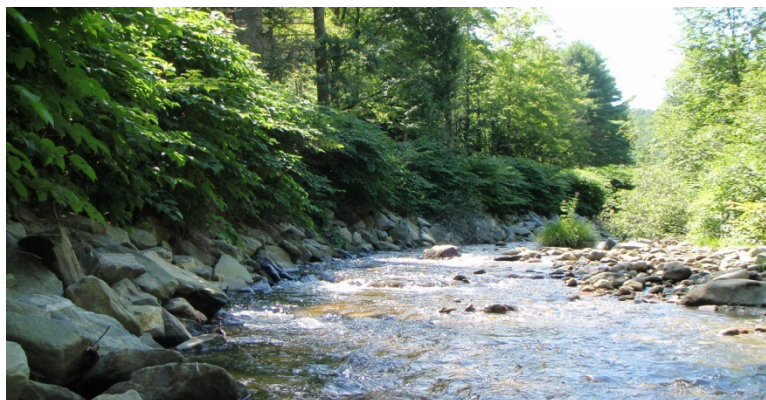
Figure 4.38 Rip-rap and road fill on the right bank
