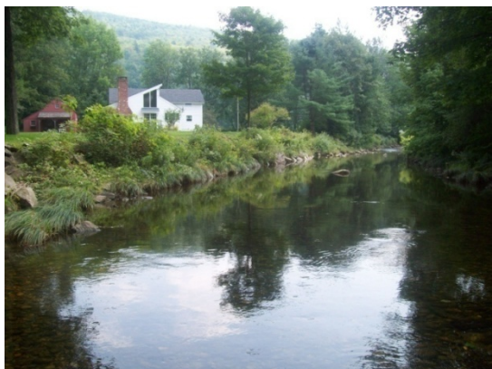
Figure 4.70 Bank armoring and development in the upper reach
