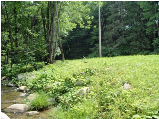
Figure 4.33 No buffer and encroachment on the left bank
