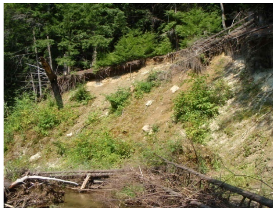
Figure 4.56 Looking downstream at the mass failure
