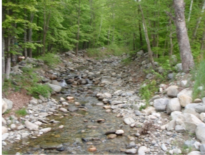
Figure 4.87 Looking upstream from the Townshend Road crossing at the dredged and straightened channel
