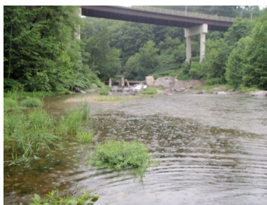
Figure 4.2 Several mid-channel bars in the widened channel
