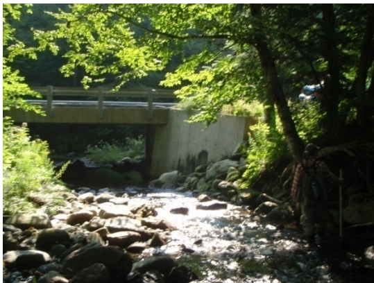
Figure 4.84 Townshend Road crossing; dredging location
