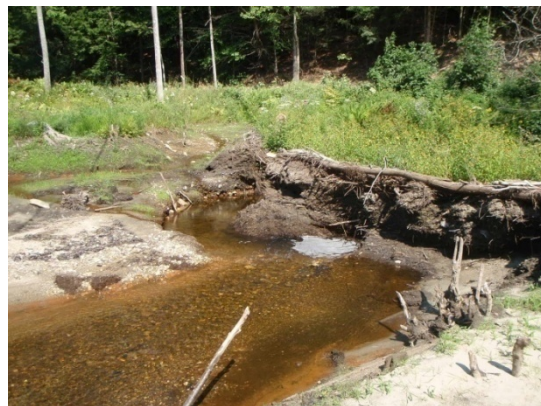
Figure 4.63 Looking downstream at the second breached dam
