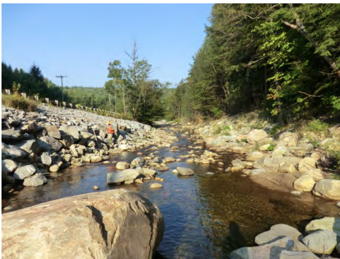
Figure 5.15. A straight, featureless channel with poor buffers dominates in T8.05-C.
