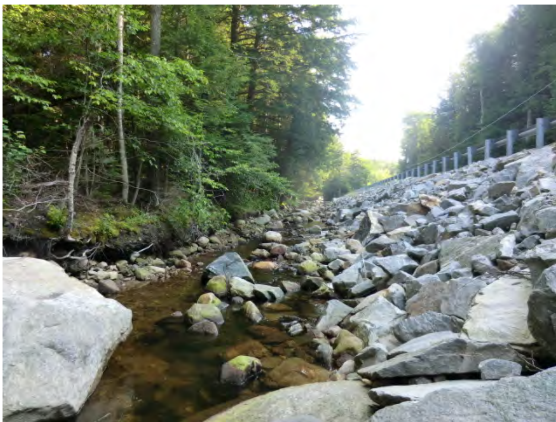
Figure 5.18. Straightened and rip rapped along the road, T8.06-C has been converted to a plane bed bedform.
