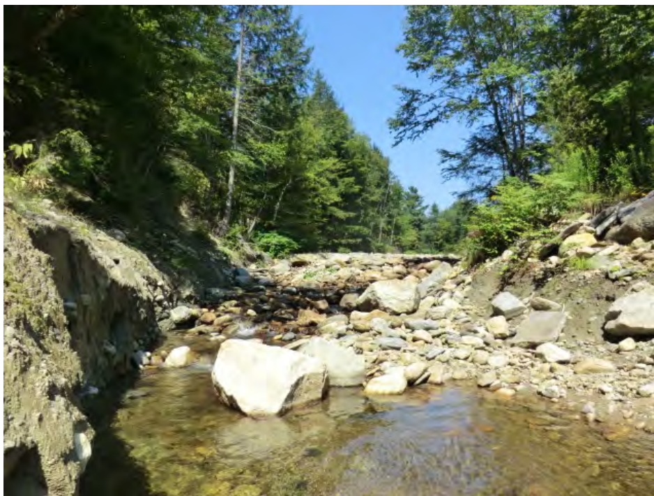
Figure 5.13. Headcut below sediment plug and high stream banks in T8.05-A.
