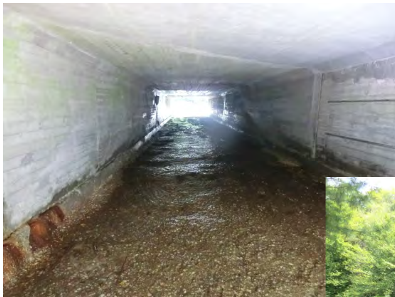
Project #28 – Culvert Retrofit
