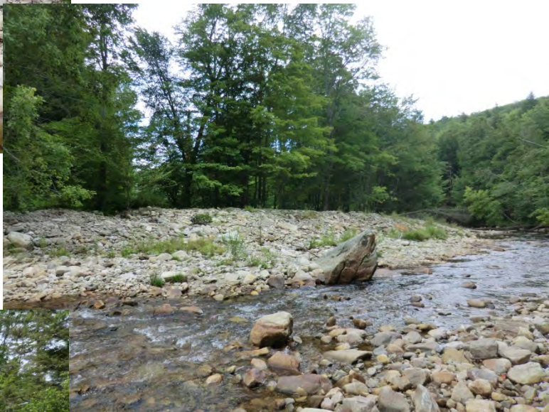
Project #16 – Return Windrowed Material to Channel & Remove Berm
