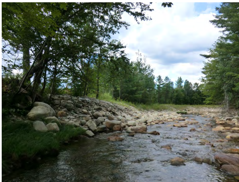
Figure 5.13. T11.06-A was windrowed extensively during post-TSI channel work and has lost its bedform.
