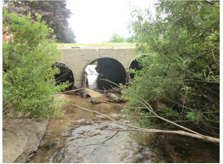
Project #30 – Culvert Replacement
