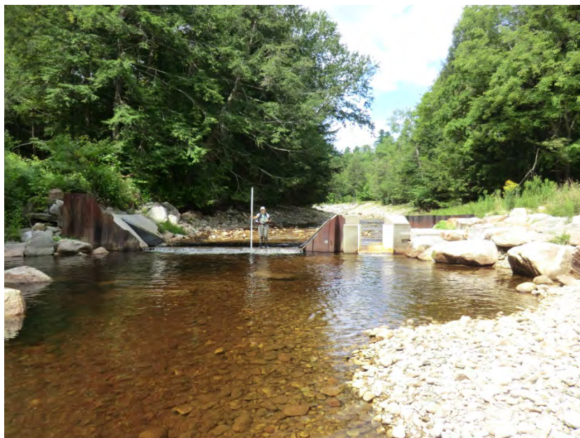
Figure 5.15. A weir in T11.07-A is impacting sediment transport throughout the segment.
