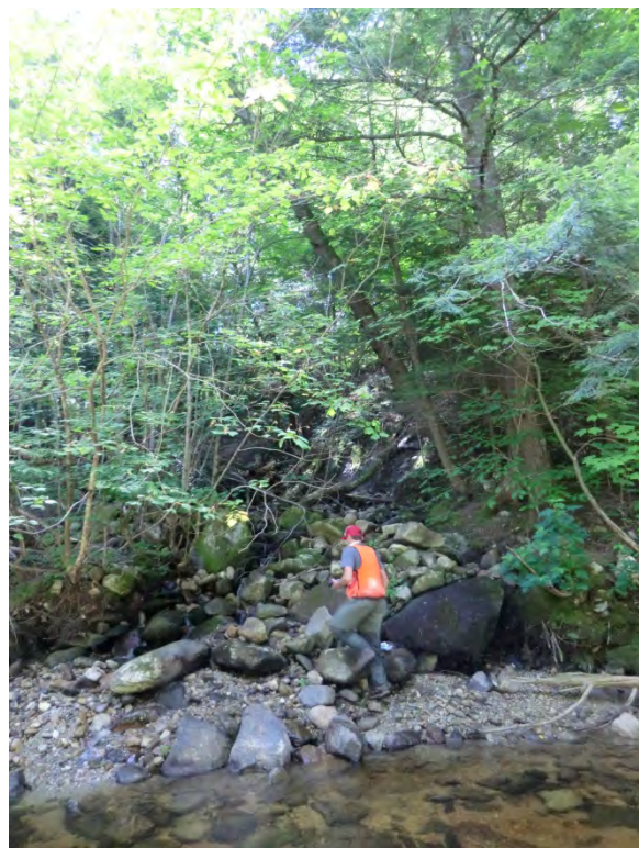
Project #18 – Remove Berm & Investigate Gully
