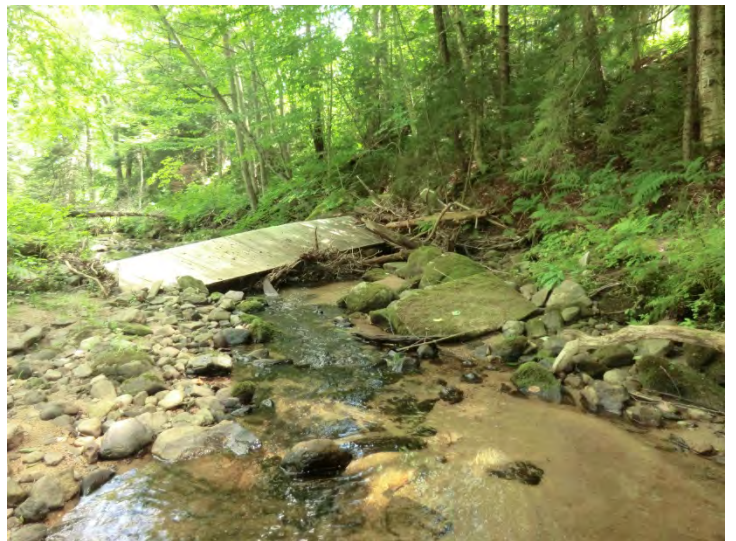
Project #32 – Remove Destroyed Footbridge
