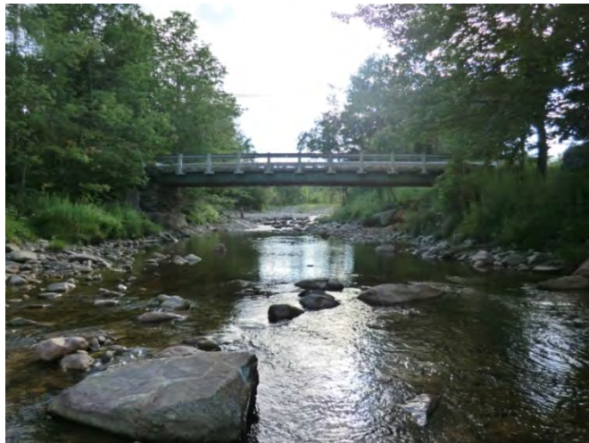
Figure 5.31. Lower Taylor Hill Rd bridge was closed at the time of assessment.
