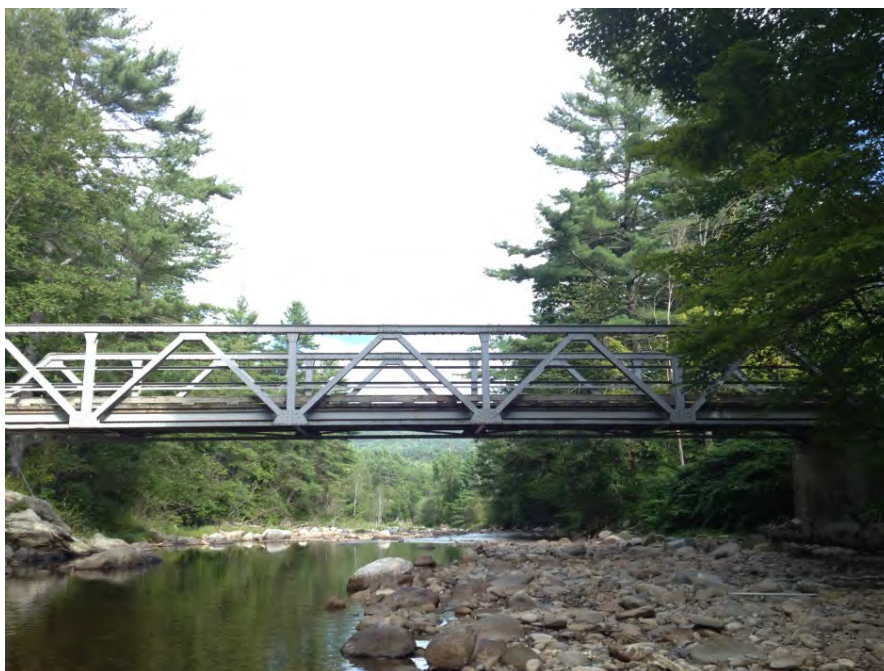
Figure 5.2. Stream crossing at the upstream end of T11.01.
