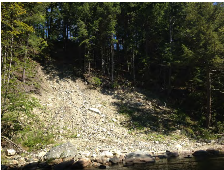
Figure 5.4. One of many mass failures present in T11.01-A.
