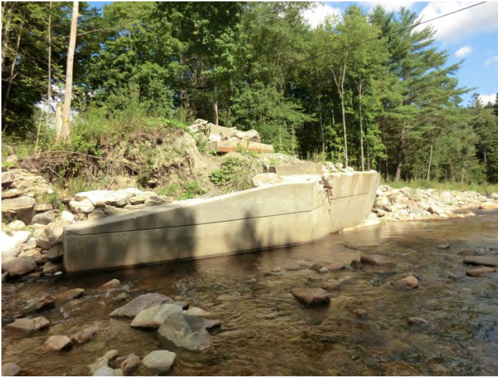
Project #3 – Remove Old Bridge Abutments
