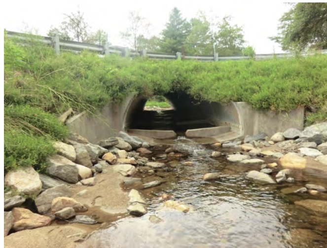
Figure 5.39. The culvert under Rt. 30 has a small drop at the outlet and baffles throughout.
