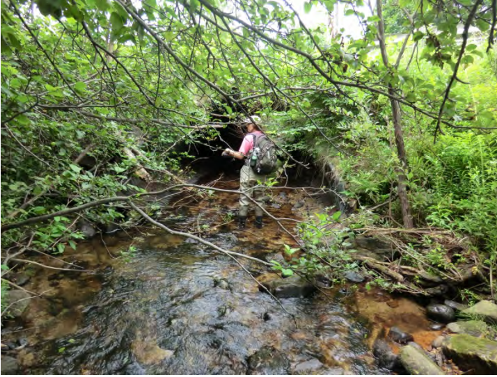
Project #29 – Culvert Replacement
