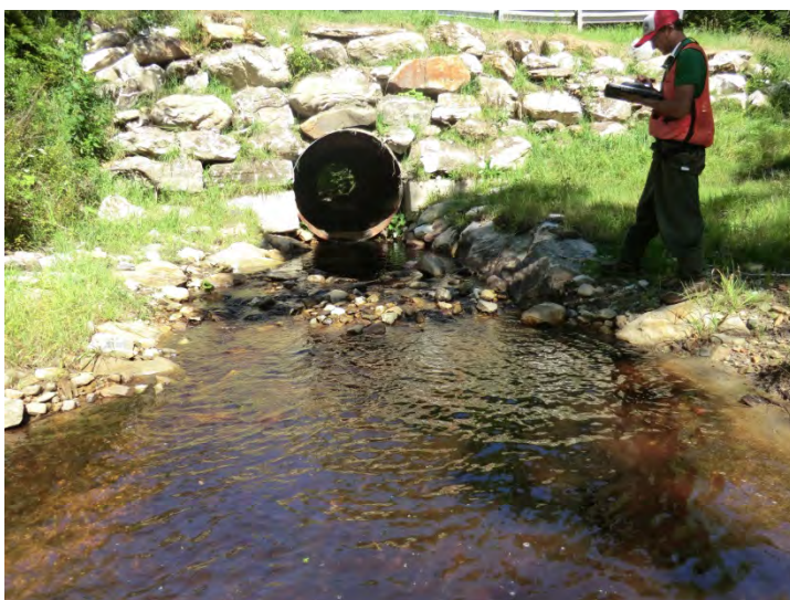
Project #28 –Culvert Replacement
