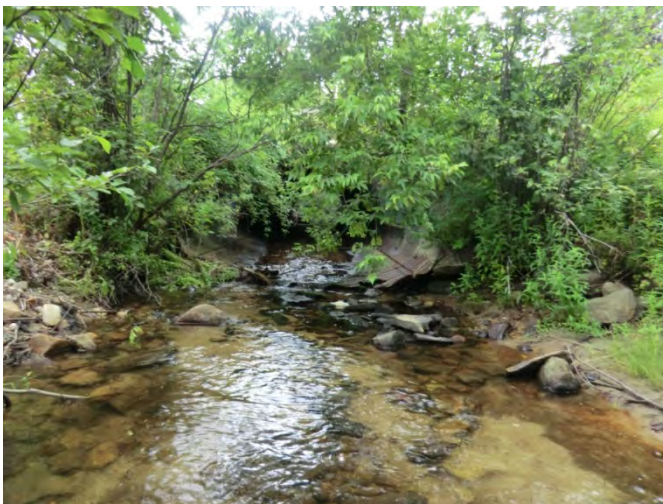
Figure 5.37. The bottom of the culvert under Rt. 30 in T11.S4.01-B is rusting out.
