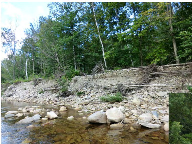
Project #15 – Return Windrowed Material to Channel & Remove Berm
