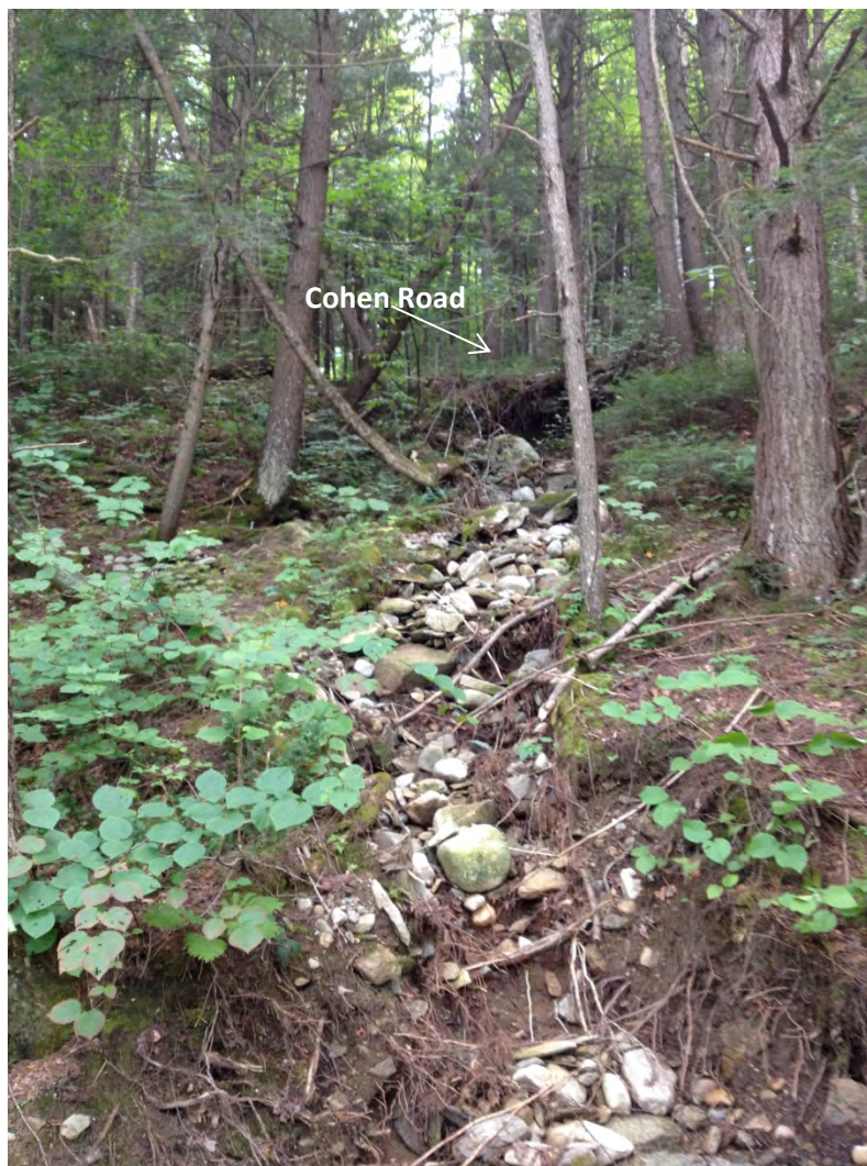
Project #2 – Stabilize/ Remediate Gully; Improve Stormwater Infrastructure
