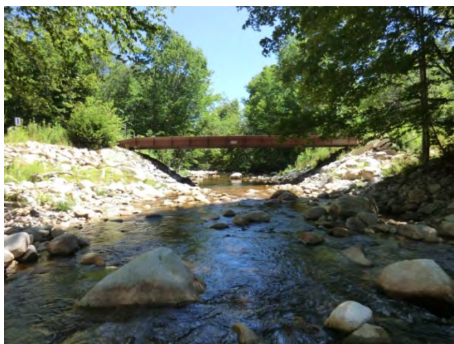
Figure 5.32. Channel constriction on Lightfoot Camp Road
