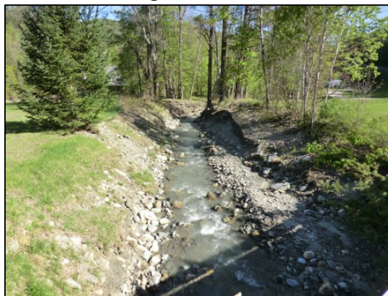
Figure 5.26. Extensive dredging and windrowing create an incised channel in R15-S1.01-A.
