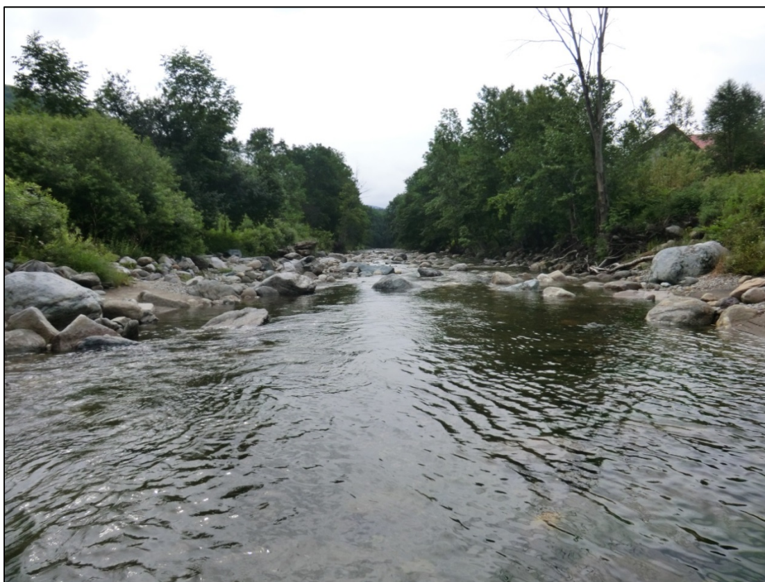
Figure 5.60. Extensive historic straightening in T7.02-E has created a featureless, plane bed channel.
