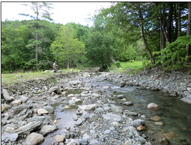
Figure 5.43. Fletcher Brook was extensively dredged and windrowed at the alluvial fan in T5.3-S1.01-A after Irene.
