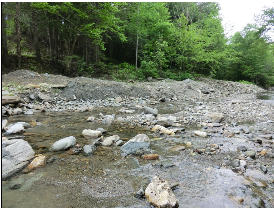
Figure 5.9. Chateauguay Road washed out during TSI in T3.03-B and post-flood work involved windrowing.
