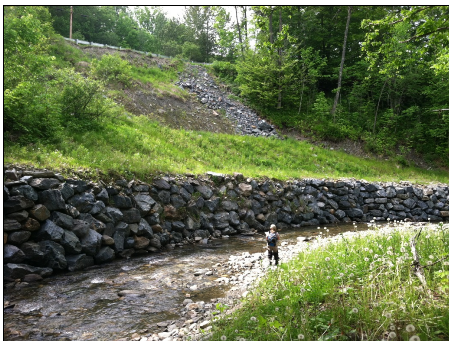
Figure 5.11. Bank instability is common in T3.04-B, as is bank armoring.
