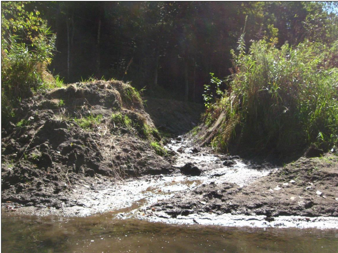
Figure 15. Freshly-dug road ditch emptying into Reach M03.
