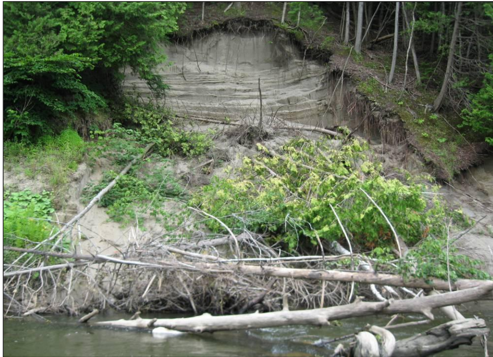
Figure 10. Example of a mass failure site, located along Reach M16.
