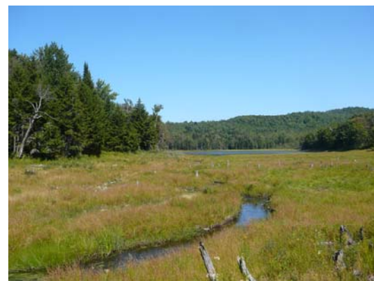
(f) view upstream from breached dam, 4 September 2009
