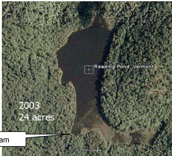
(a) Reading Pond prior to 2006 dam breach.
