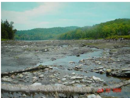
(e) view upstream from breached dam, 22 June 2006 (Source: VTDEC).
