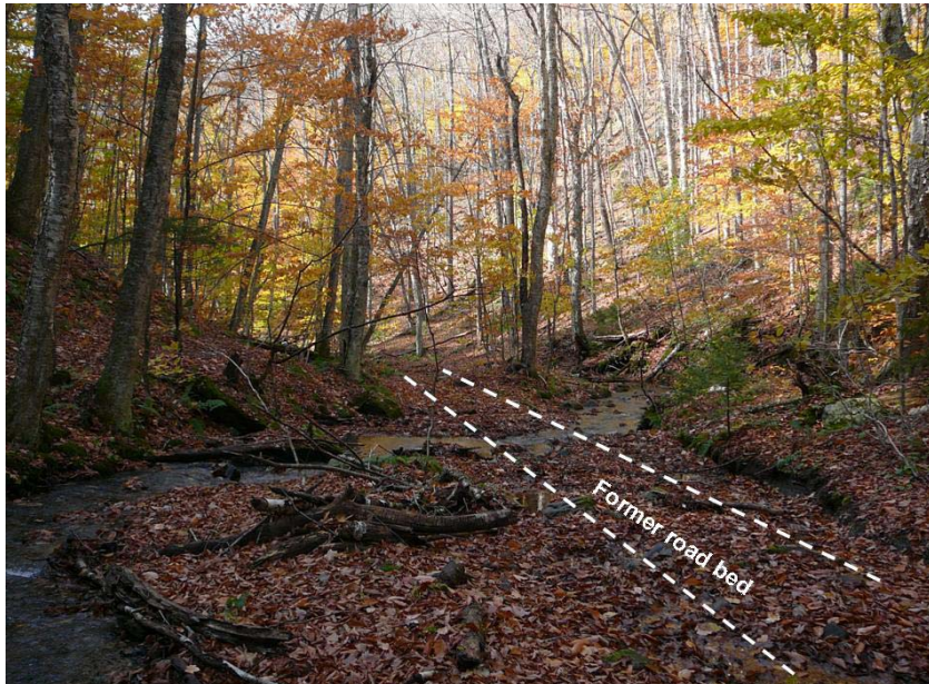
Figure 20. View downstream, river crossing old road bed, which now functions as a flood chute during higher-flow conditions upstream of the crossing, Segment A, reach M41T6.05, Buffalo Brook, 22 October 2009
