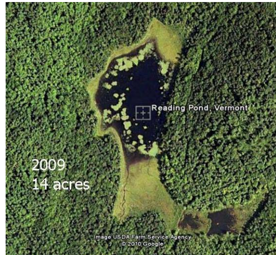
(b) Reading Pond after 2006 dam breach.
