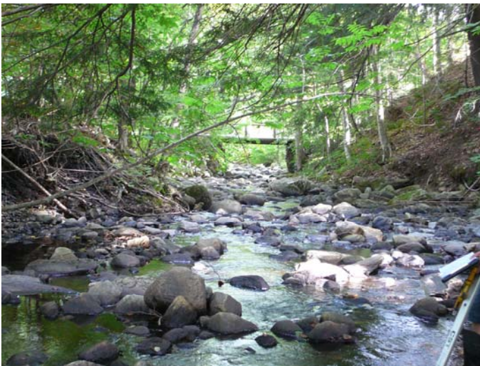
Figure 16. View downstream to Library Road bridge, M40T5.01 Segment B, Patch Brook; 10 September 2009
