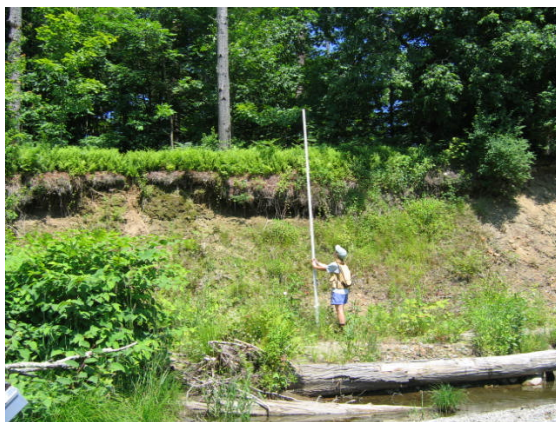
Figure 7.39. Mass failure 20 feet high along eastern bank in Reach T4.01
