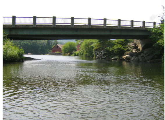
Figure 7.11. Bridge at Moscow Road in Reach M11
