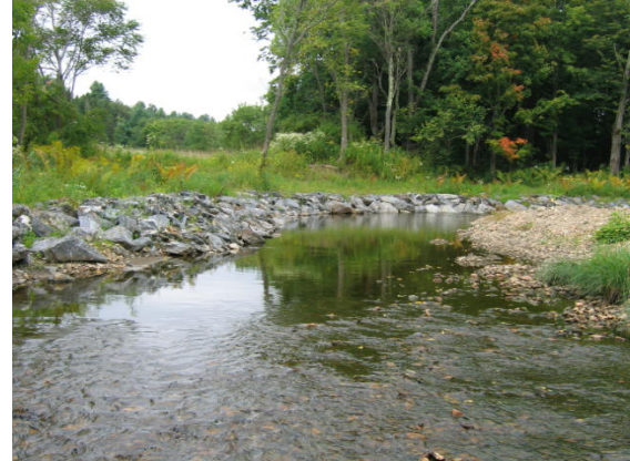
Figure 7.34. Rip-rap along bank upstream of Tansy Hill Road Bridge in M20
