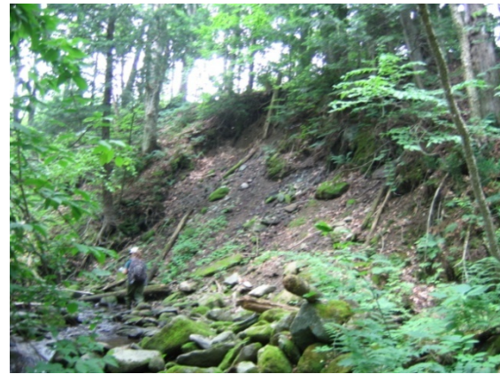
Figure 7.62. Mass failure in T6.07
