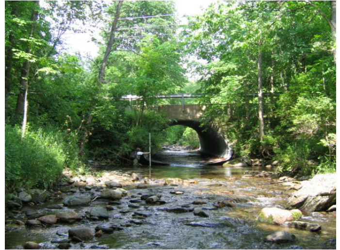
Outlet – invert is freefall
