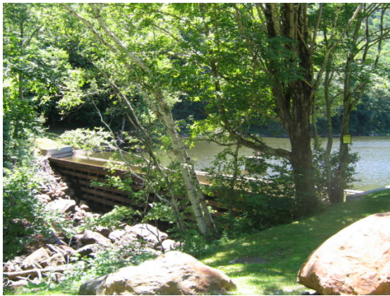
Figure 7.47. Lake Mansfield Trout Club dam at upstream end of T4.05
