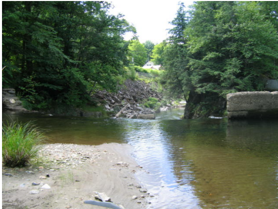
Figure 7.22. Old dam grade control is constricting channel and causing sediment deposition upstream in M15-A.
