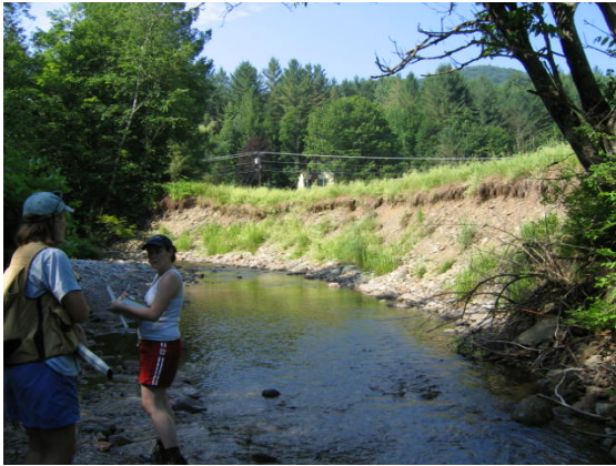
Figure 7.37. Lack of buffer along western bank causing bank failure in Reach T4.01
