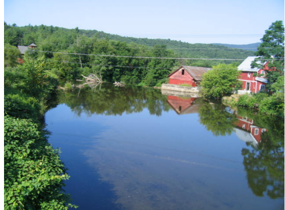
Figure 7.12. Moscow Mills Dam in Reach M11
