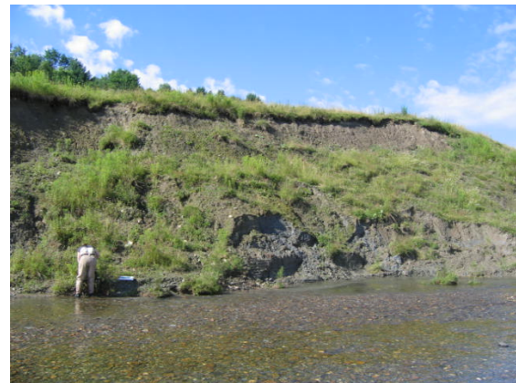
Figure 7.64. Mass failure acting as a major sediment source in Moss Glen Brook in T8.01-B
