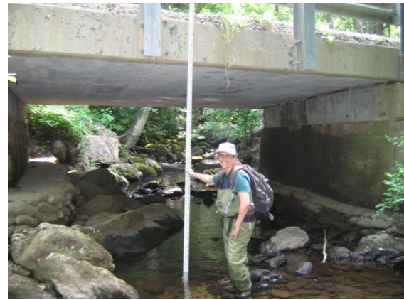
Figure 7.48. Constricting bridge at Nebraska Valley Road in Reach T4.05
