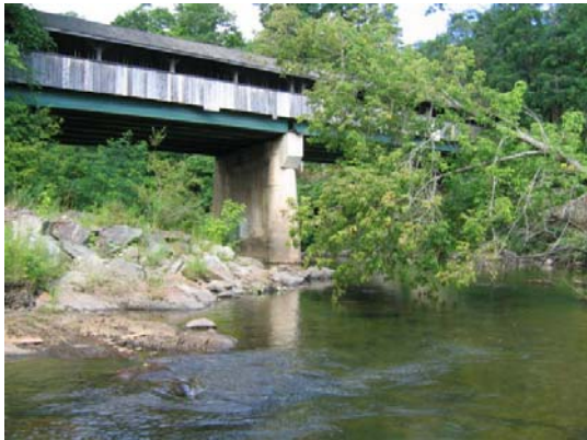
Figure 7.25. Route 108 bridge at downstream end of Segment M15-D
