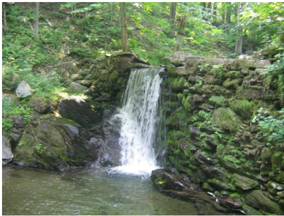
Figure 7.61. Old rock dam grade control in T6.07
