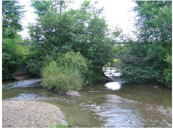
Outlet – at grade
