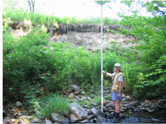
Figure 7.38. Mass failure 12 feet high along western bank in Reach T4.01
