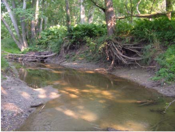
Figure 1. M01 bank erosion near outlet
