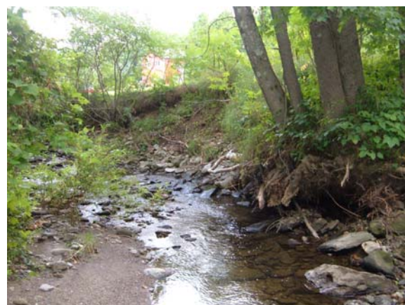
Figure 14. Bank erosion in upper M06
