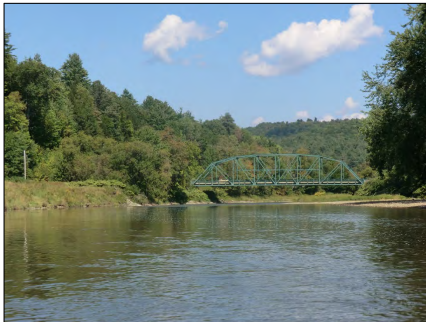
Figure 5.10. Development is prevalent along the Winooski River in R13 (Winooski Street Bridge pictured).
