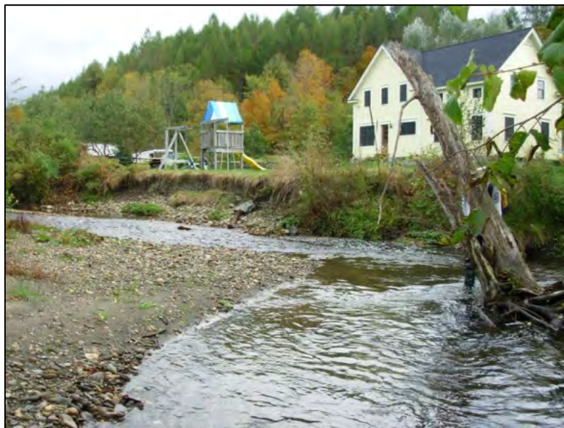
Figure 5.31. River corridor encroachment and lack of riparian buffer in R13.S1.02-S1.04-A.
