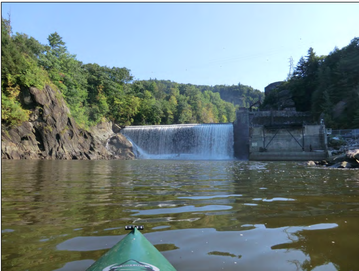
Figure 5.8. M2.01 impacted by valley width changes by placement of I 89 and Route 2 bridges.
