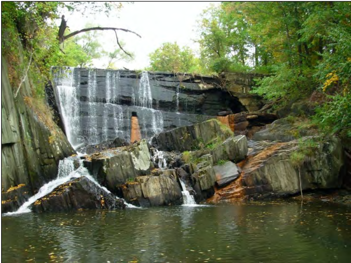
Figure 5.26. R13.S1.02-S1.01-B flows through a bedrock gorge that has two dams in it.
