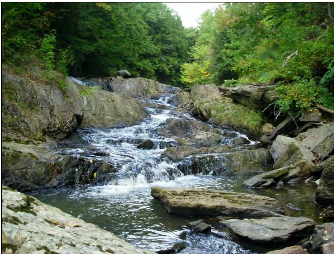
Figure 5.20. R13.S1.02-A is a bedrock gorge and is very stable.
