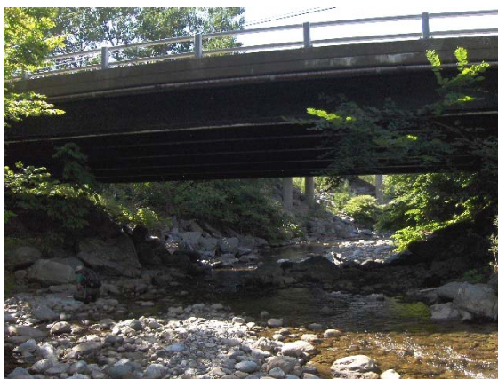
Figure 14. Route 2 bridge with reduced span.
