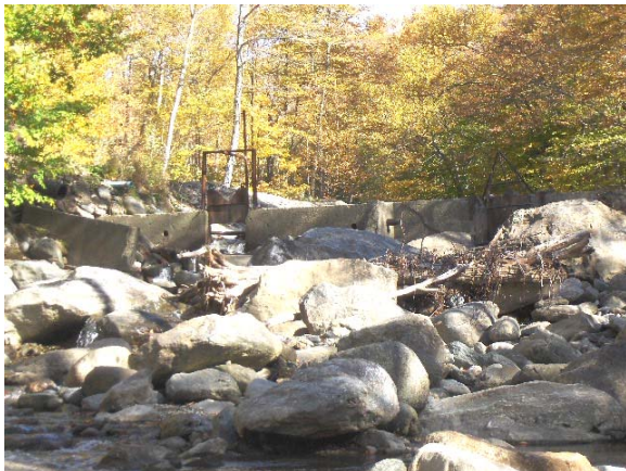
Snowmaking weir in R10.S3.04-C
