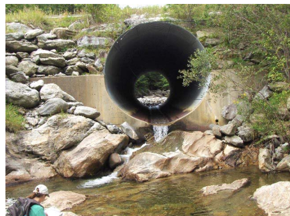
Figure 15. Bolton Valley Access Rd. Culvert
