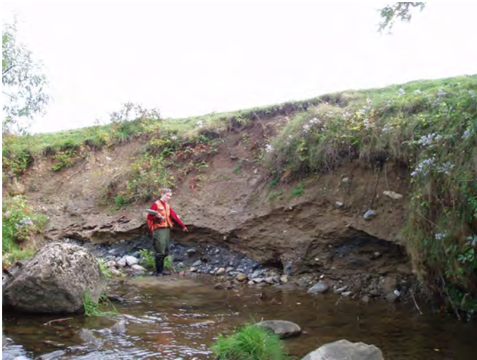
Figure 12: Rugg Brook M02- Mass Failure with Undercut Bank
