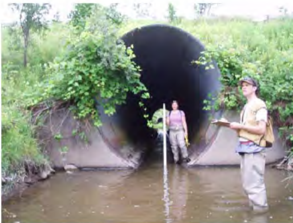
Figure 18: Deer Brook M03A- Major Culvert
