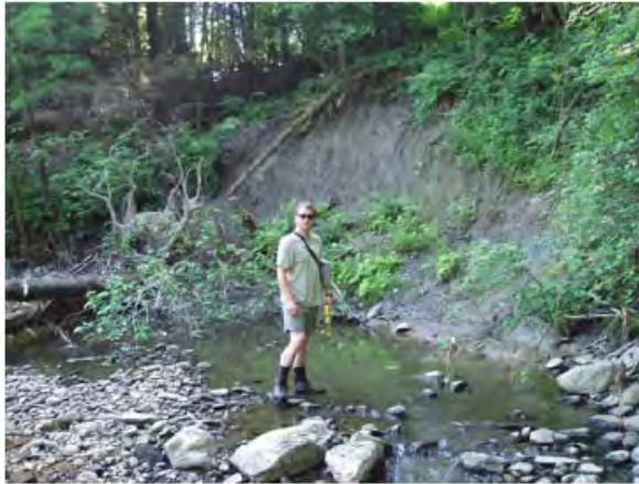
Figure 6: Deer Brook M02- Mass Failure
