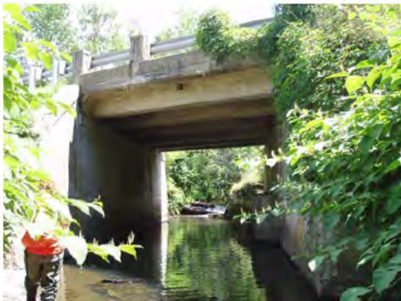
Figure 19: Mill River M05- Ethan Allen Highway Box Culvert
