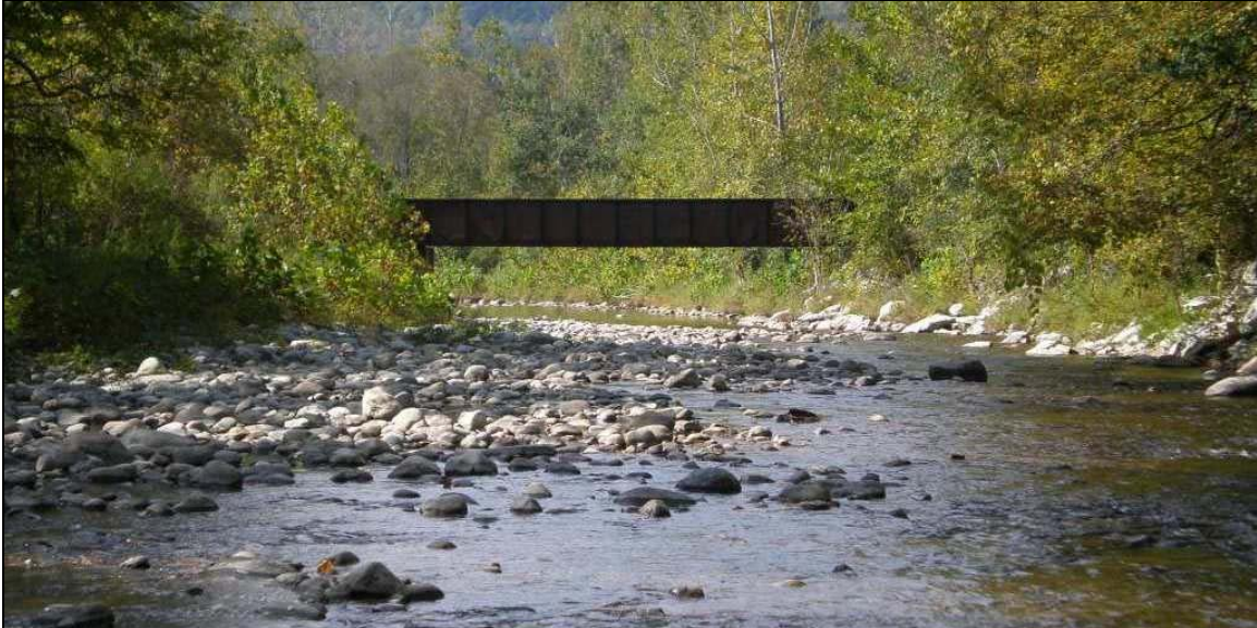
Figure 31. M01-B has been significantly impacted by channel straightening, berming, dredging, and armoring.
