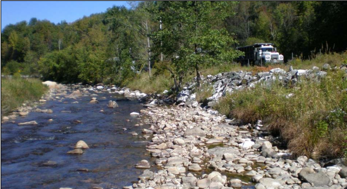
Figure 21. M06 flows through Cuttingsville and has been significantly impacted by channel straightening, armoring, berming, and floodplain development.
