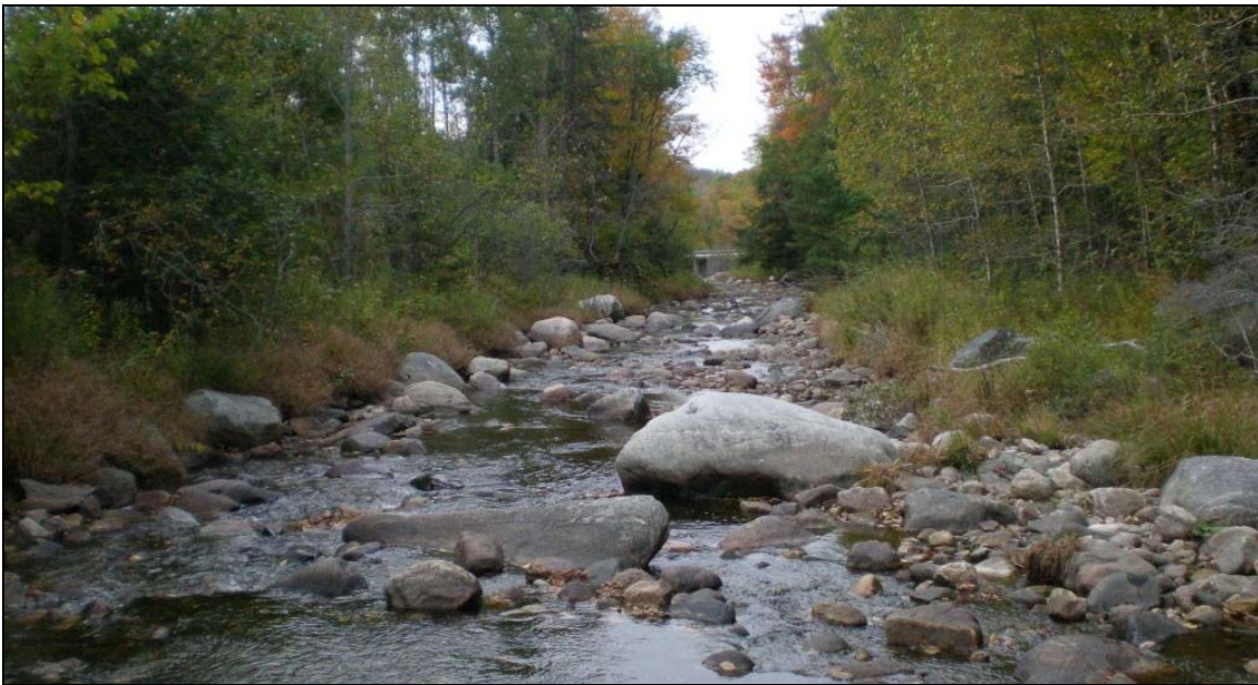
Figure 8. M14 has been historically straightened and is now has a plane bed form. Widening and planform adjustment are actively occurring.
