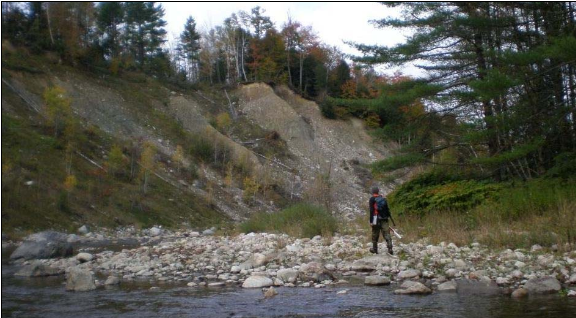
Figure 24. A large mass failure on the left bank is providing some sediment recruitment to help rebuild bars in the incised Mill River reach M05-A.
