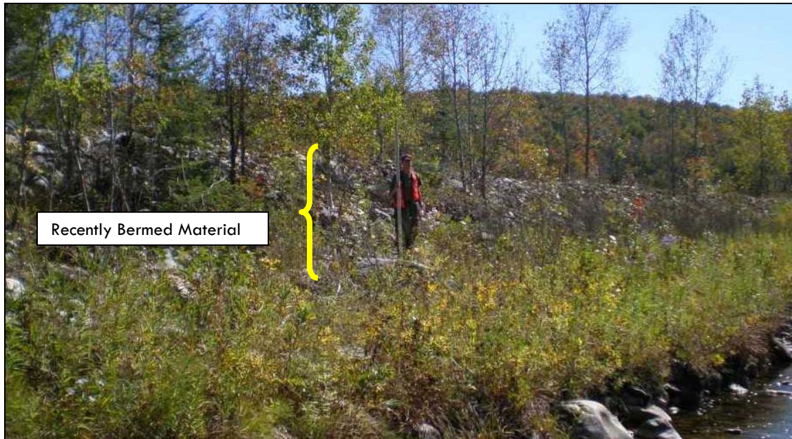
Figure 20. M07 has seen significant berming on the right bank causing a significant loss of floodplain access.
