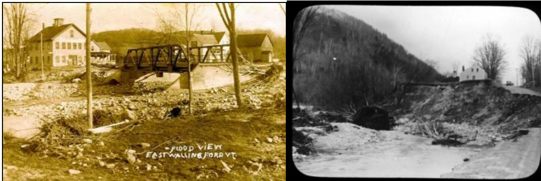
Figure 3: These image shows damage from the 1927 flood. Left image is looking towards the intersection of Route 104 and Route 155 (Reach M10) in East Wallingford. Right image is of route 103 washout in Cuttingsville near reach M06/M07.
