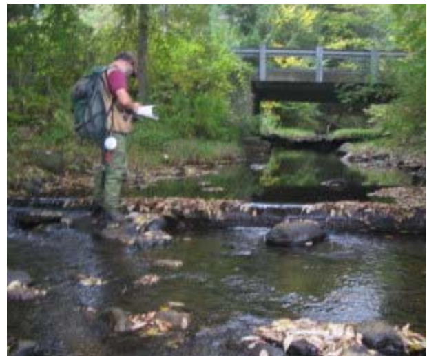
Figure 31. Segment M04-T2.01B had better buffers but lacked the bedrock grade controls present downstream in this reach. The check dam in this photo may have been installed to limit upstream migration of headcuts and bed degradation.
