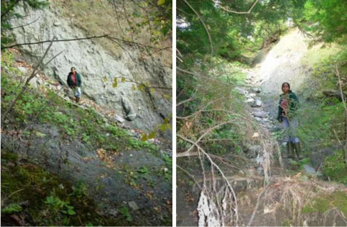
Figure 26. Mass failure/gully in M03-T1.02A appears related to a one-time break in a water line upslope of the stream near Dutton Hill Road.
