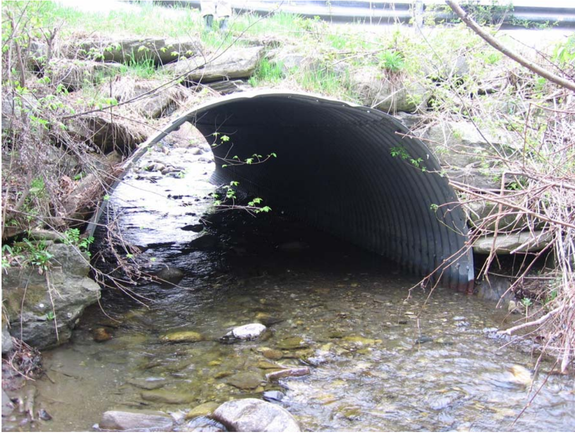
Figure 5 – Natural bed, at grade, Turnpike Road & Upper Turnpike intersection
