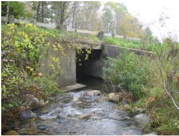
Figure 42. Bridge alignment and the presence of a driveway above the right bank (right side of this photo) combine to form both a stream channel and a flood-prone constriction in segment M08B.
