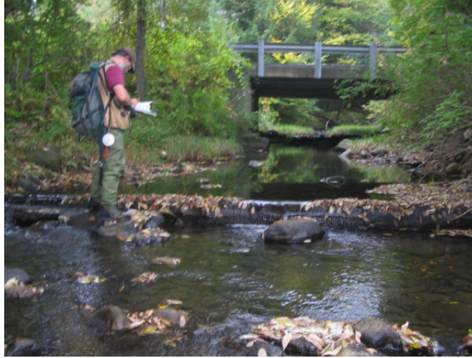
Figure 11. The check dam in this photo was likely installed to limit upstream migration of headcuts and bed degradation below the Norwich Pool impoundment, indicating sensitivity of the stream to the “sediment starving” resulting from retention of sediments above the dam in reach M04-T2.03.
