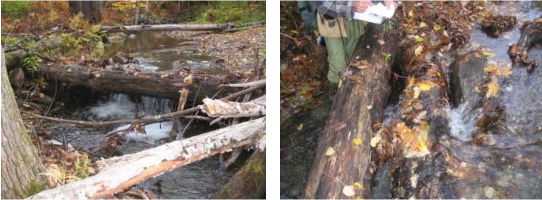
Figure 43. A log dam in segment M08C (left) that appears to have been installed as part of a stream ford to access a log landing has been eroded and is now forming an active headcut with the potential to migrate upstream rapidly (right).
