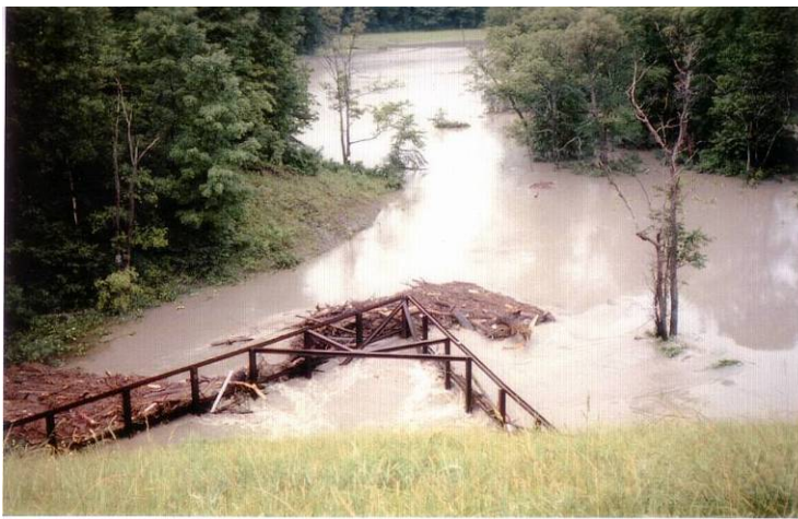
Figure 6. Photos from 1973 show floodwaters rising up the embankments at Rte. 5 (also shown in Fig. 5) , as well as the damage caused at the Beaver Meadow Rd. bridge just north of the Norwich village center (photos courtesy of Andy Hodgdon).
