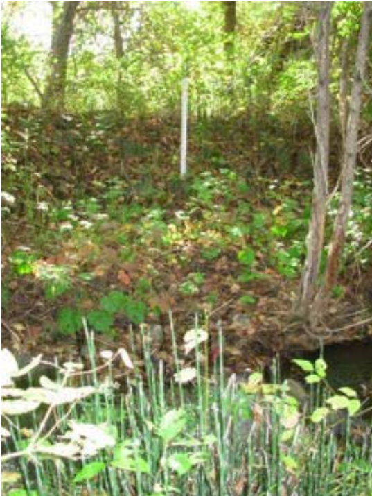
Figure 50. A high berm on the left bank of segment M03-T1.01A prevents the stream from accessing the floodplain.
