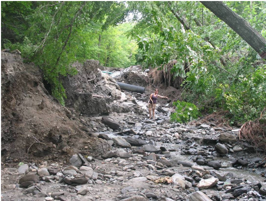
Figure 55. This road was taken out by a small, unnamed tributary of Ayers Brook in Randolph, Vermont, when the stream avulsed and cut a new channel in an intense thunderstorm during July 2007. The woman at the center of the photo is indicating the post-flood width of the stream by her armspan.
